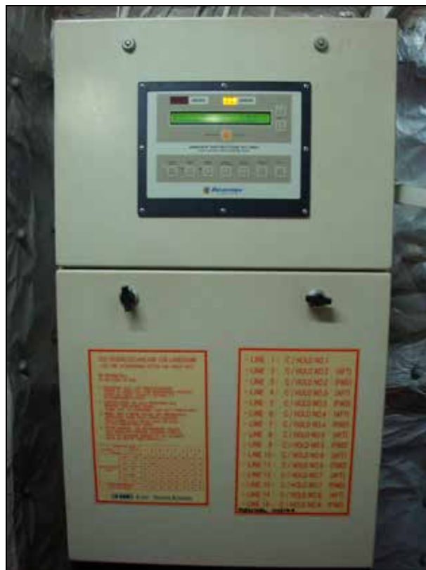
Figure 8: Identical sample extraction smoke detection system (MSC ALESSIA)
