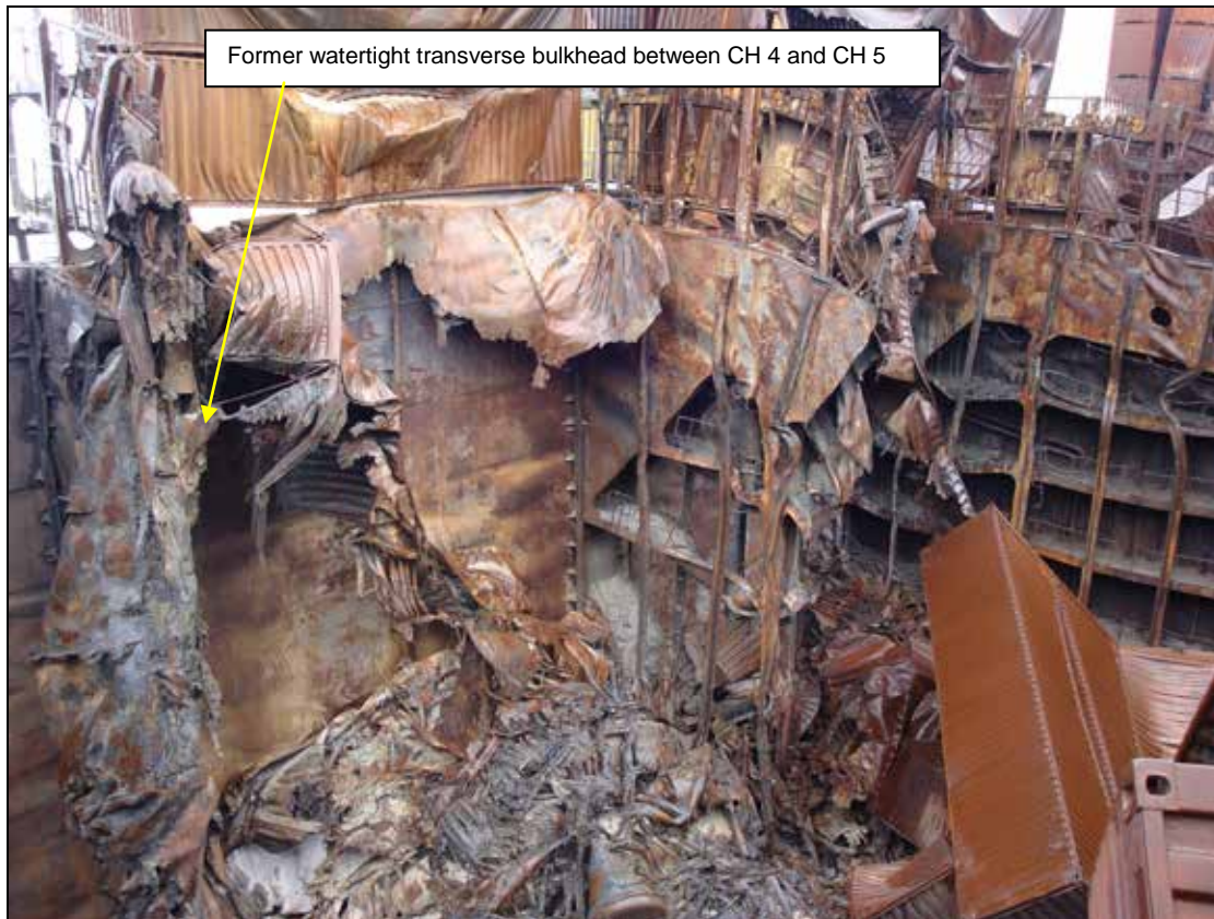
Figure 31: View through cargo hold 5 up to transverse bulkhead to cargo hold 6
