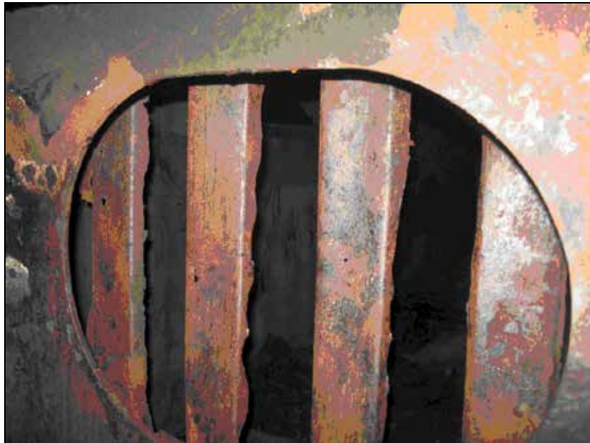
Figure 26: Ventilation opening in a container in cargo hold 3
