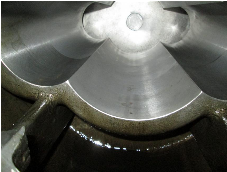
Figure 32: Pump body after removing the spindles
