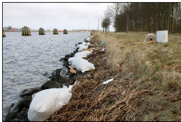
Figure 22: Flotsam, cargo damage
