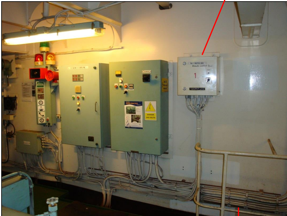
Figure 11: Switch cabinets for the steering gear
