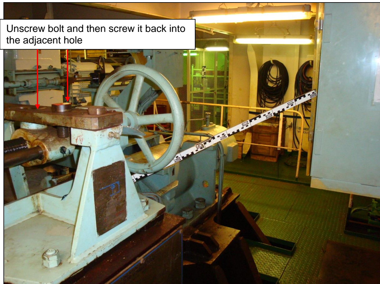
Figure 13: Switching to manual emergency operation
