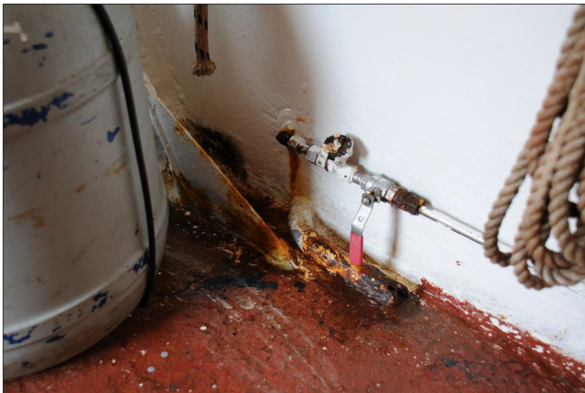
Figure 5: Main ball valve with upstream throttle needle valve
