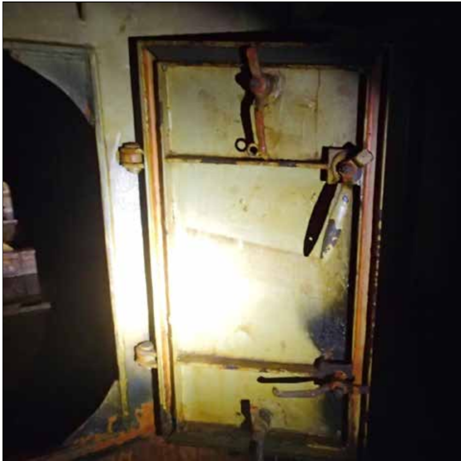
Figure 15: Internal door (bulkhead)
