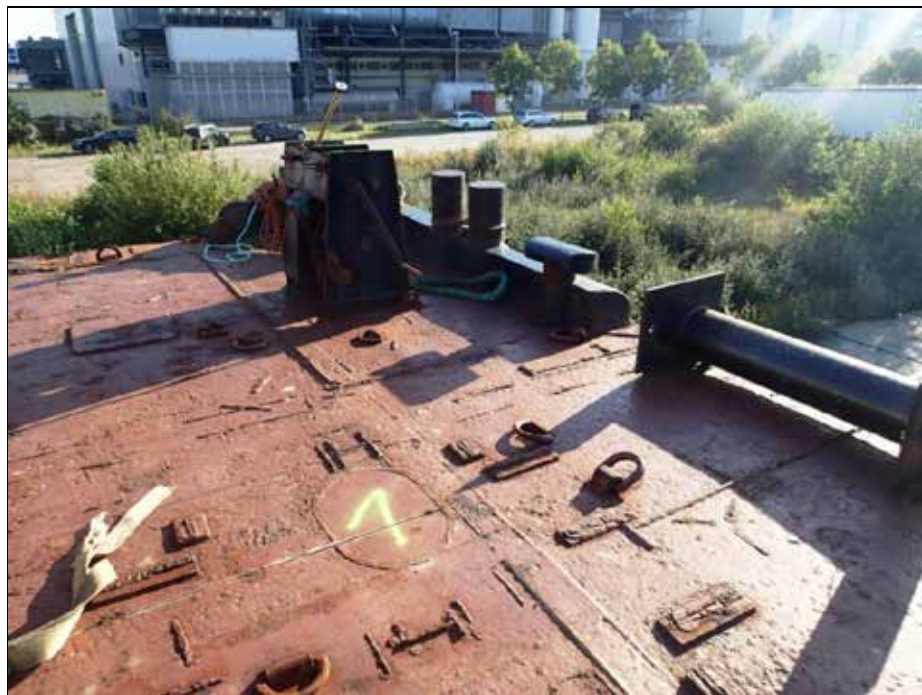
Figure 16: Example of a manhole welded closed
