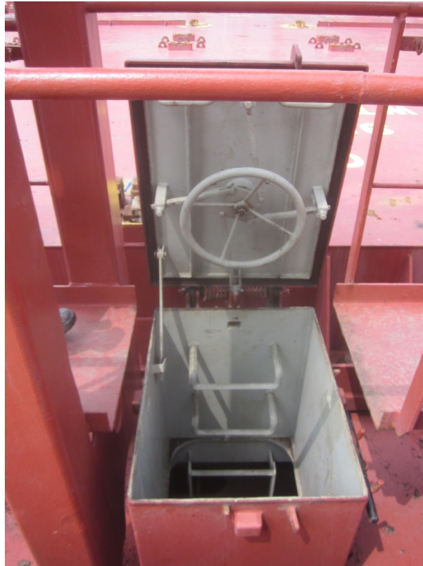
Figure 5: Access to cargo hold 9 from the main deck
