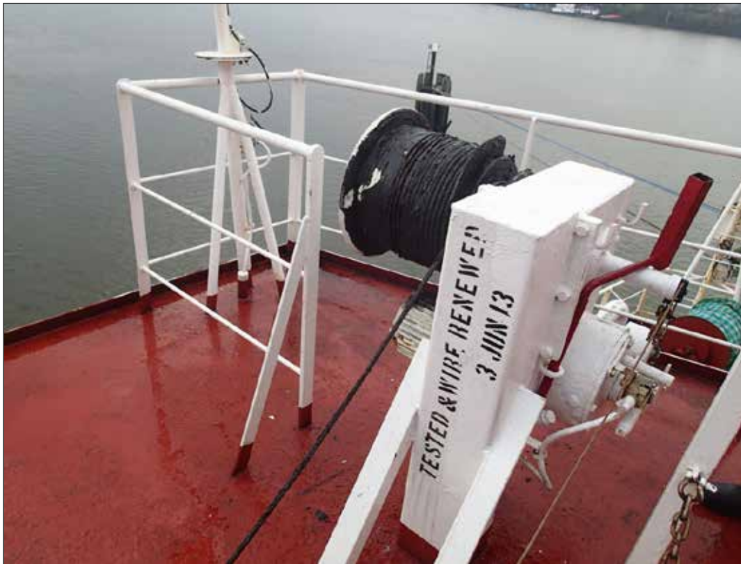
Figure 13: Winch marked with the last cable replacement
