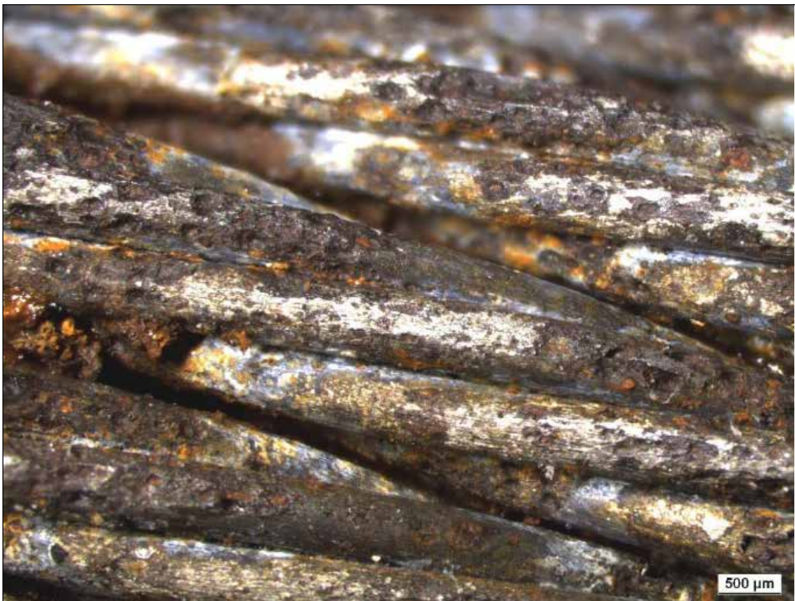
Figure 27: Corroded surface of the cable after being cleaned with kerosene
