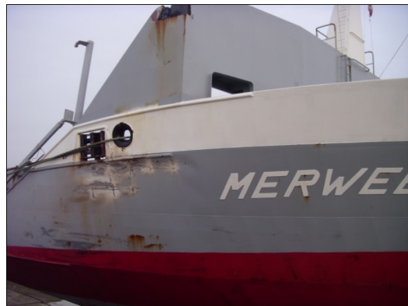
Figure 5: Bow damage on the MERWEBORG
