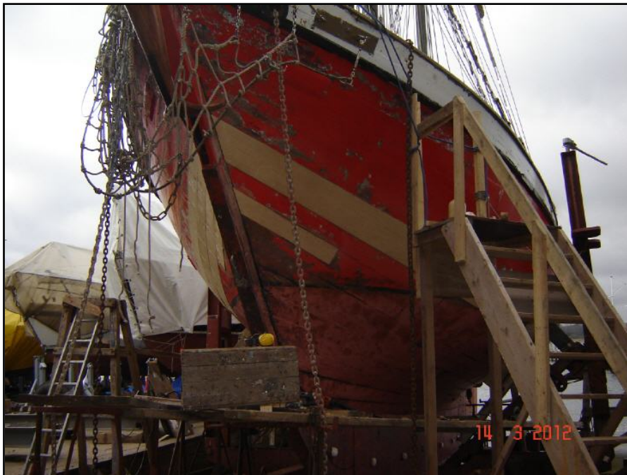
Figure 4: Renewed planking on the port side
