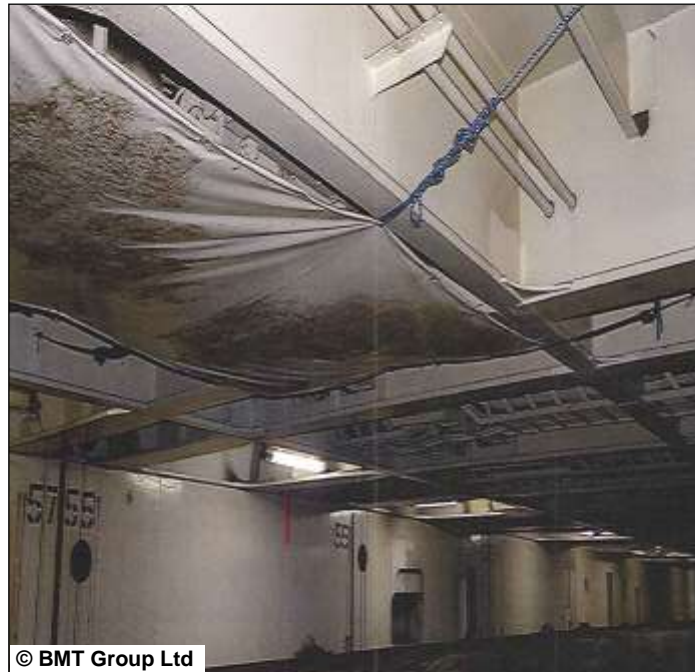
Figure 75: Example of one of the tarpaulins beneath the cargo hold ceiling
