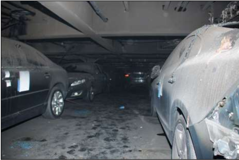
Figure 49: Spread of fire by convection (not depending on the position of the seat of fire)
