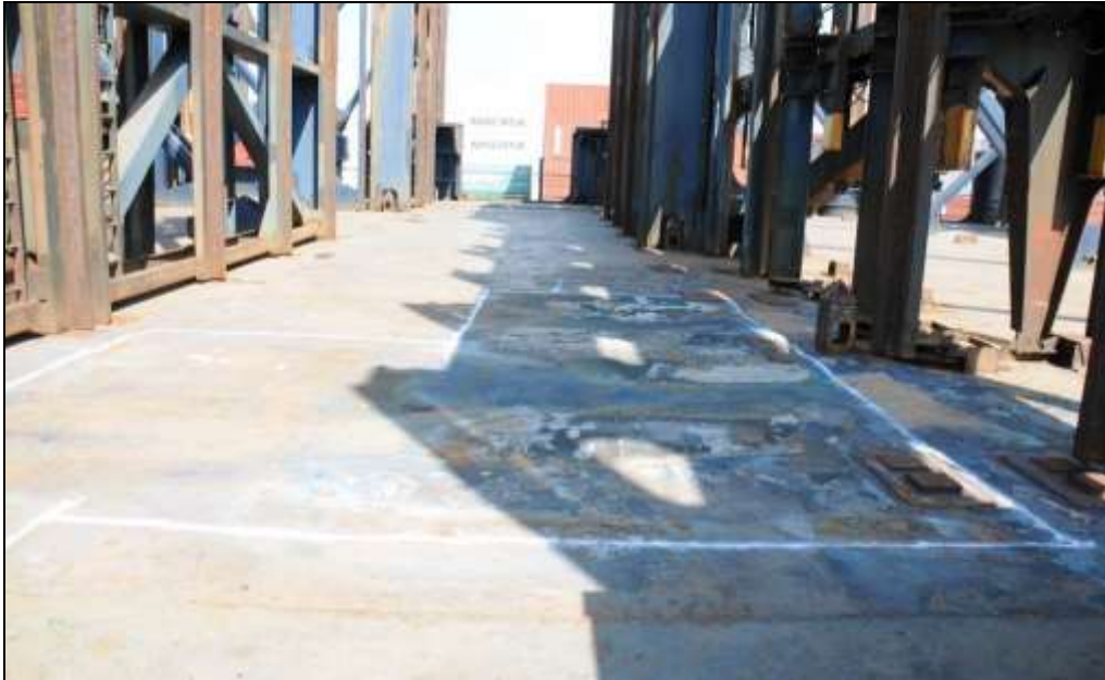
Figure 6: Heat-induced discolouration and deformation on the floor of the main deck
