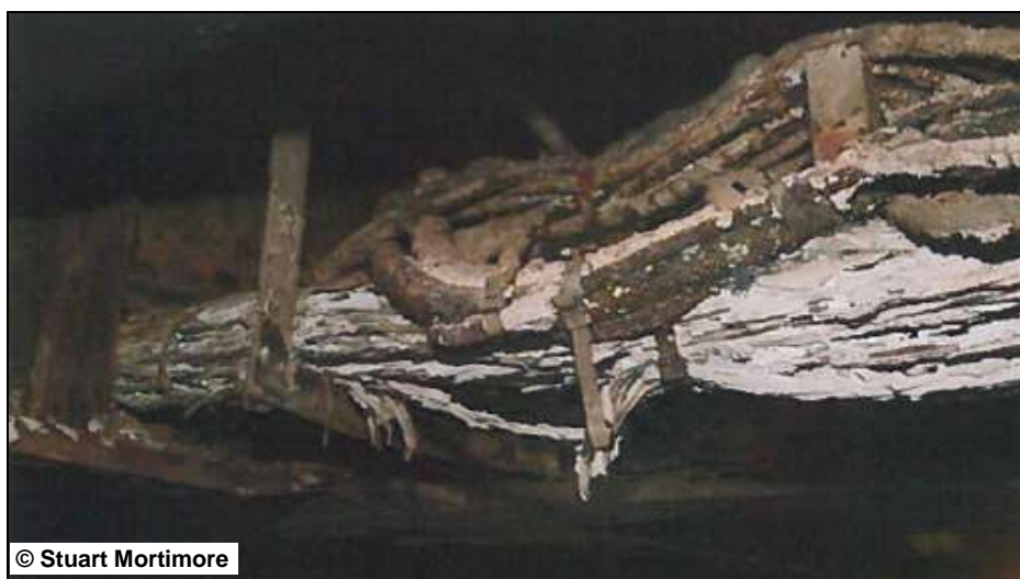
Figure 80: Cable splice above vehicle 5 B 53
