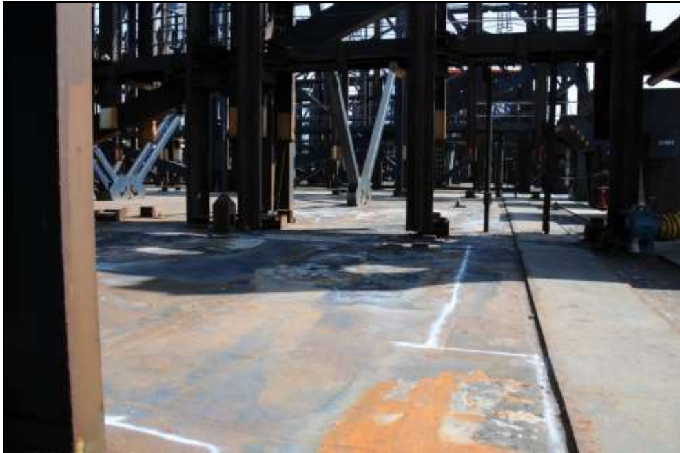
Figure 57: Damage threshold (cargo hold/void space)
