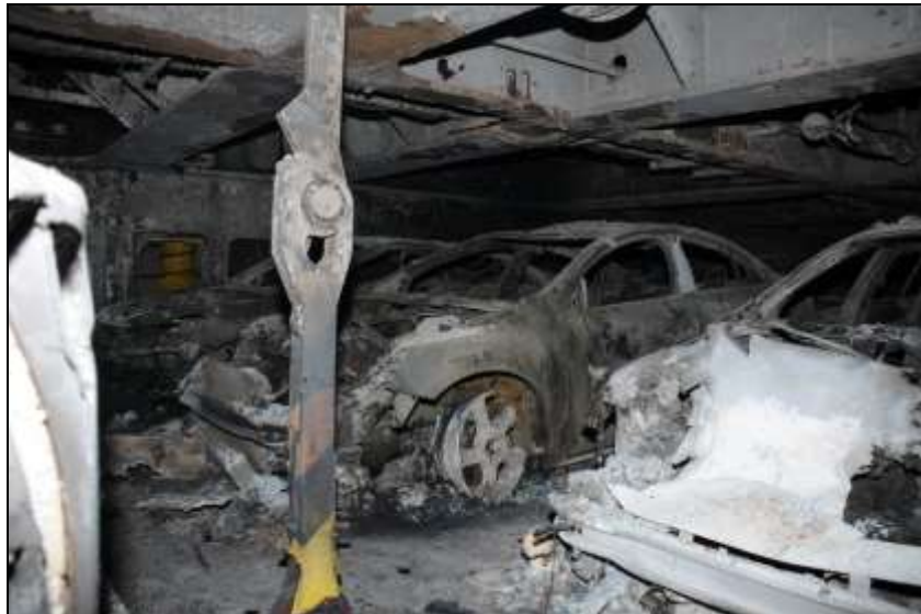
Figure 44: Apparent position of the seat of the fire (bay 26)
