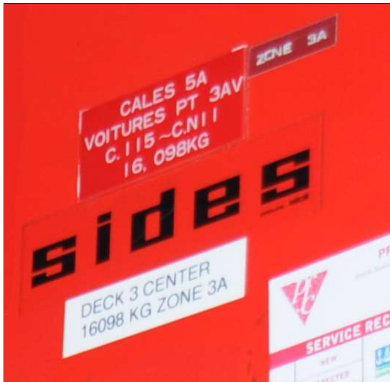
Figure 23: Close-up of the signs on the control box for zone 3 A
