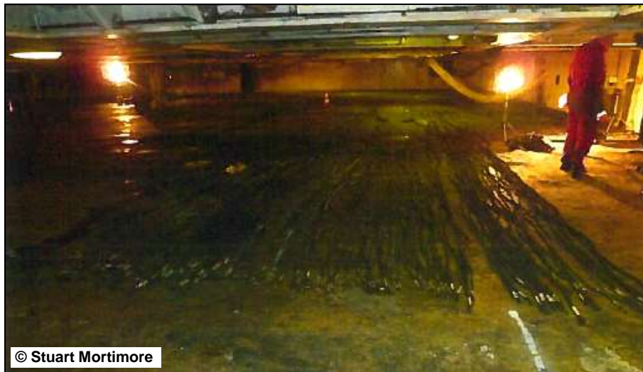
Figure 79: Example of dismantled cable harnesses 52
