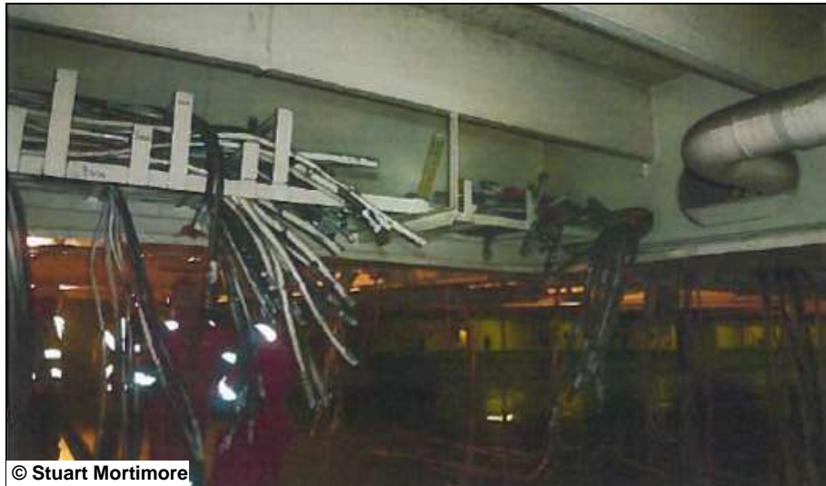
Figure 81: Rear cable splice 54
