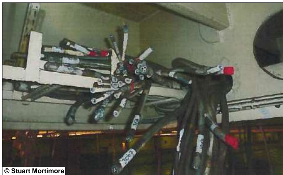
Figure 82: Cable marked for repair purposes 55
