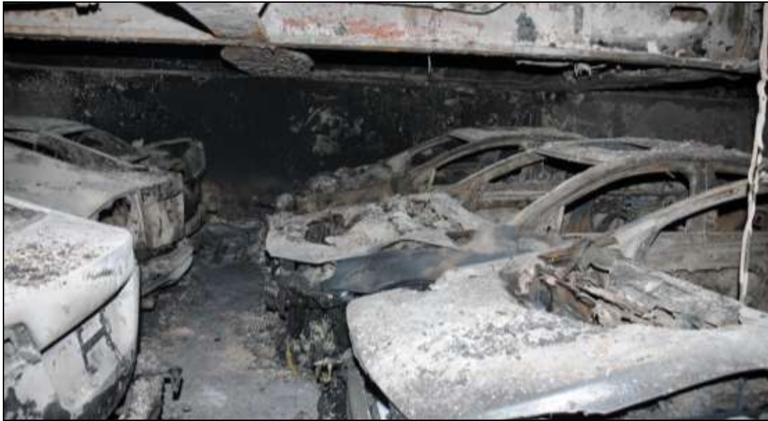
Figure 7: Completely burnt out vehicles on deck 3 B
