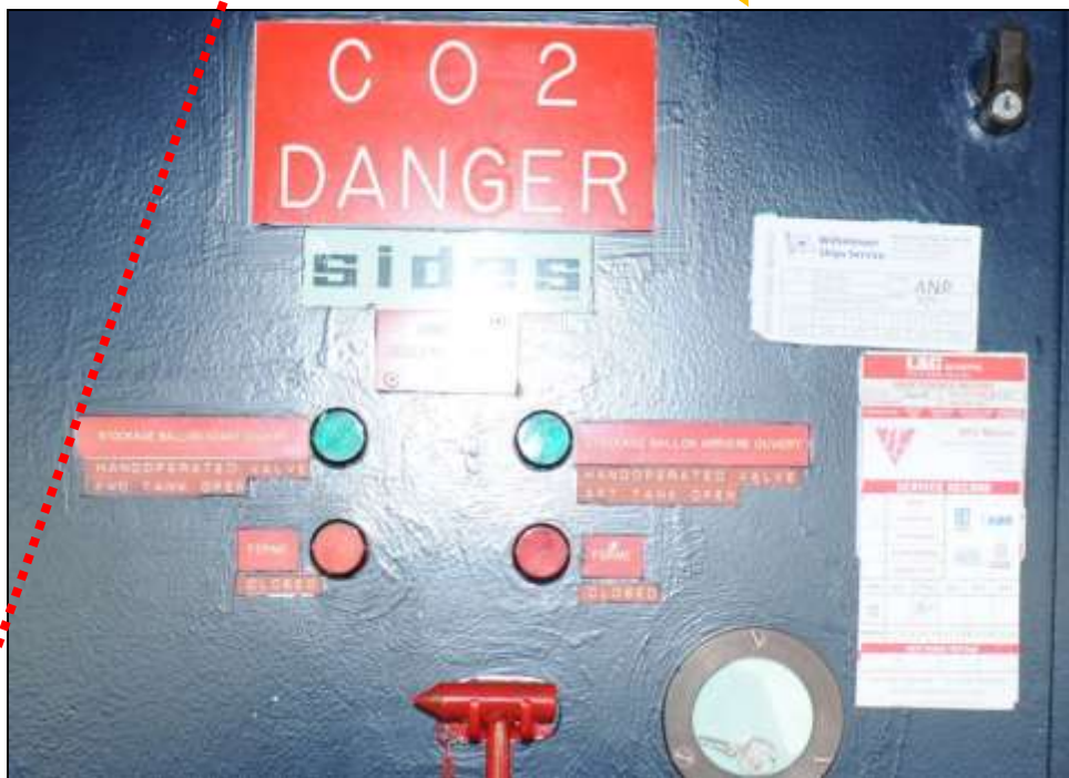
Figure 19: Extract showing the CO 2 installation controls
