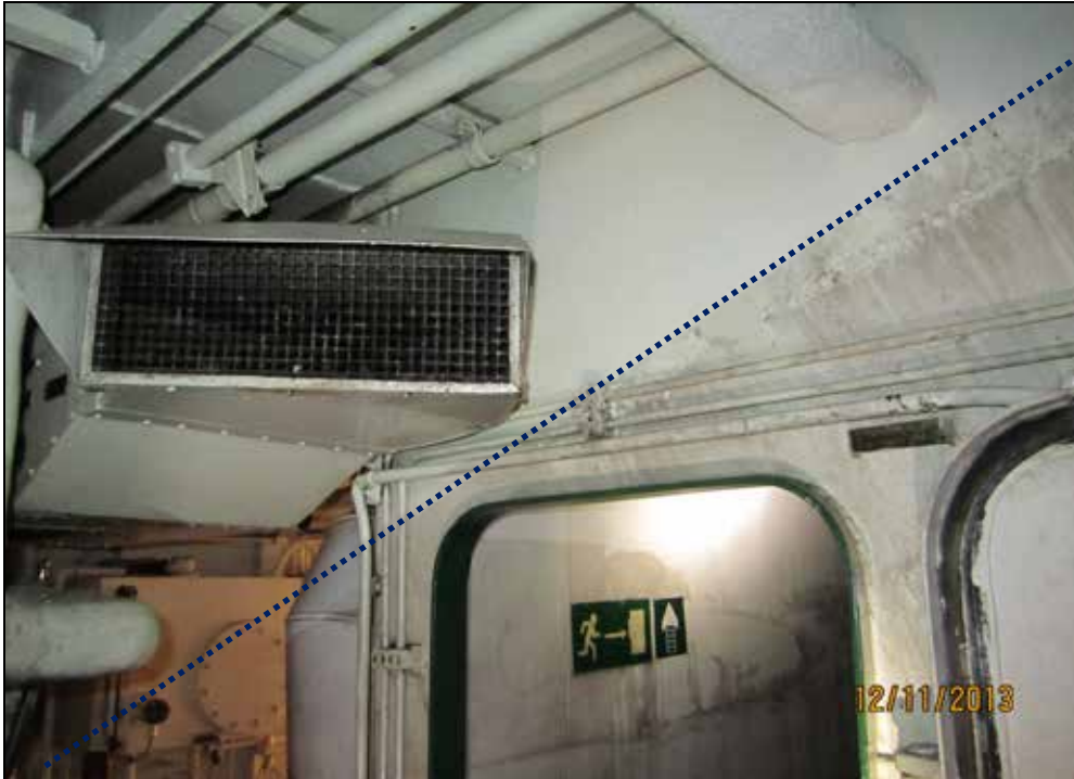
Figure 45: Evidence of the increasing flooding towards the port side of the engine room
