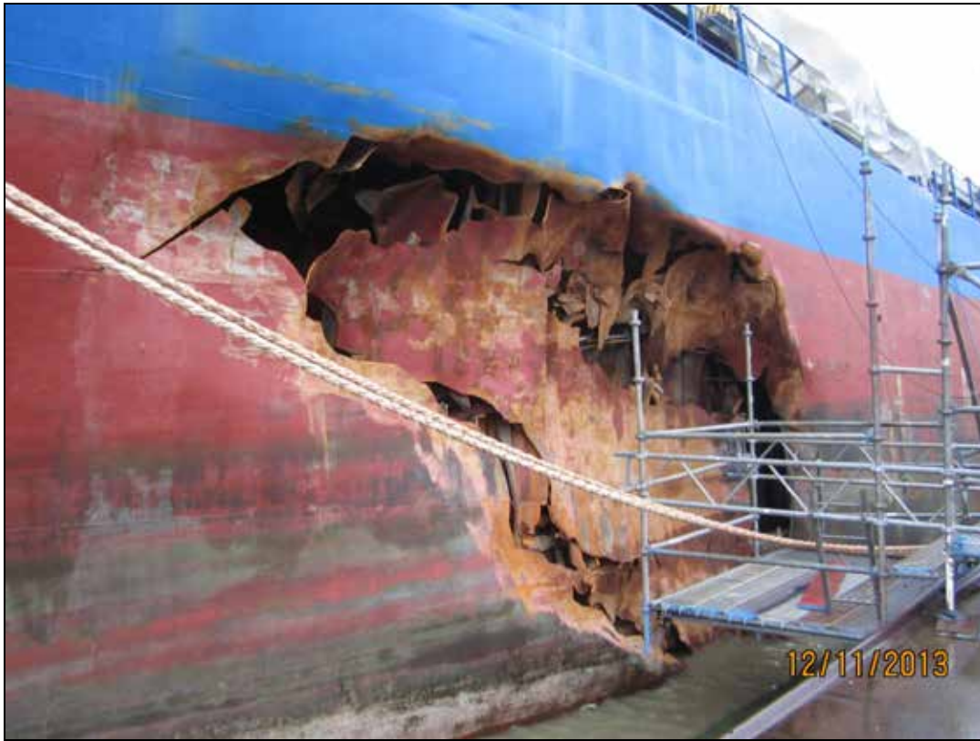
Figure 9: Hole in the SIDERFLY's hull (port side)
