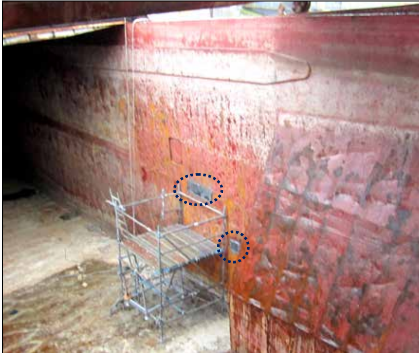
Figure 43: Holes in the cargo hold bulkhead (cargo hold 1 on port side) 30
