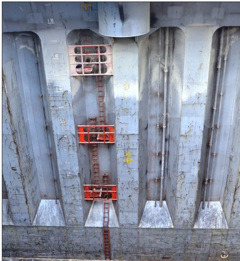
Figure 5: Vertical steps at the aft edge of CH3
