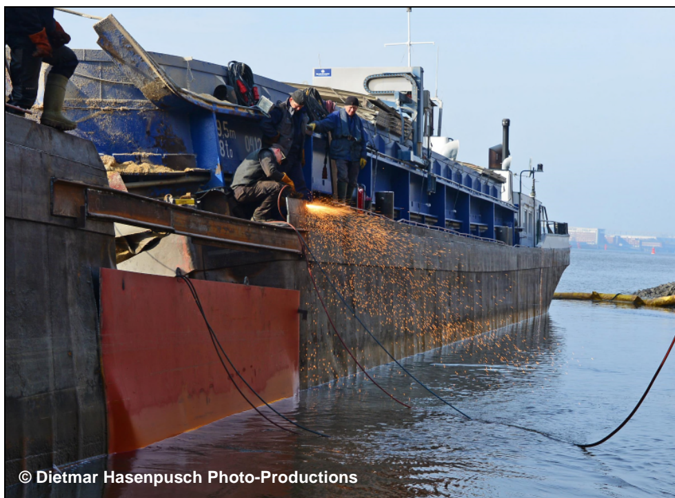
Figure 20: Leakage repairs on the JADE
