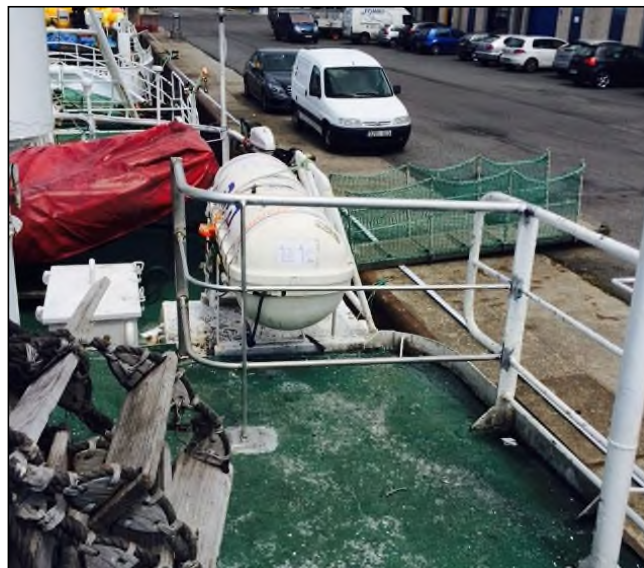
Figure 4: View of the guard rail after the modification
