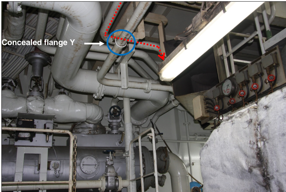
Figure 9: Routing of the discharge pipe (close-up C)
