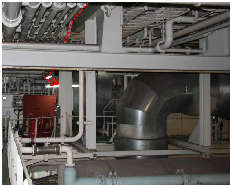
Figure 5: Upper section of the engine room in the ship's transverse direction 6
