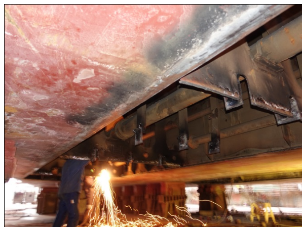
Figure 5: Damage to the bottom
