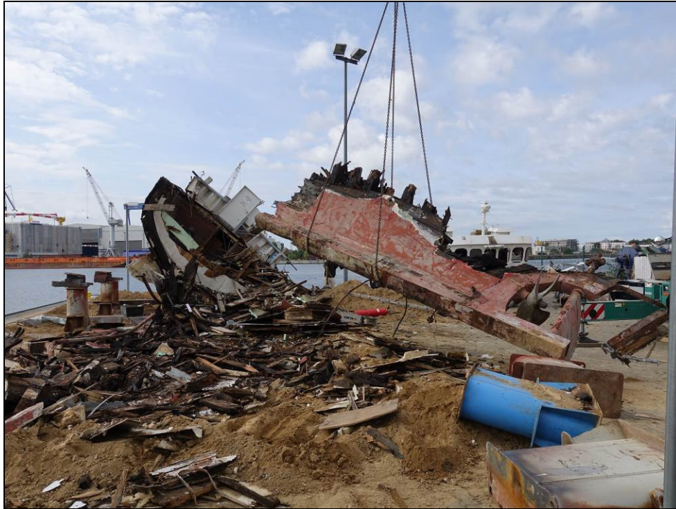
Figure 17: Scrapping the FV CONDOR at the buoy yard (final phase)
