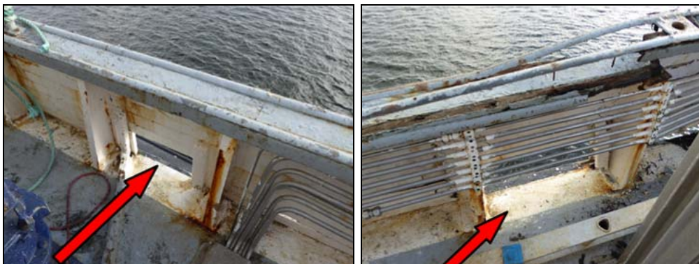
Figure 110: Freeing port openings on the port side
