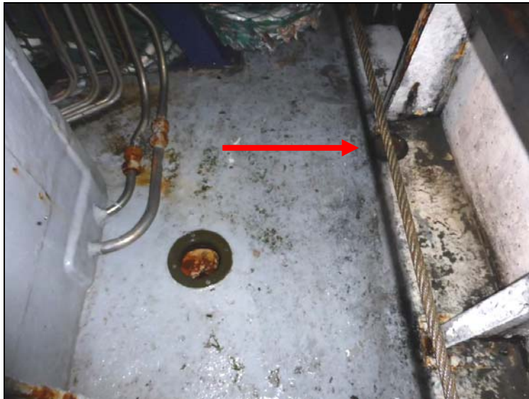
Figure 19: Opening 2 in the main deck (the associated cover is at the top right)
