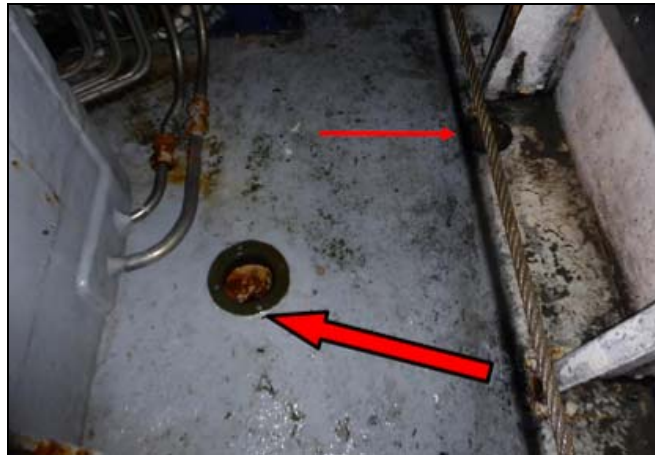
Figure 105: Tank opening on the starboard side
