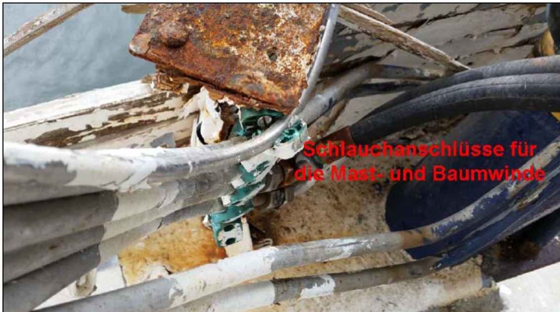
Figure 103: Destroyed hoses and pipes on the port railing
