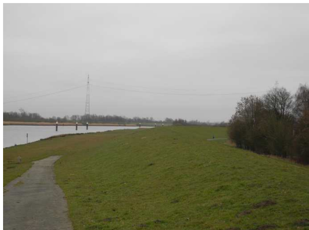
Figure 5: High-voltage power line
