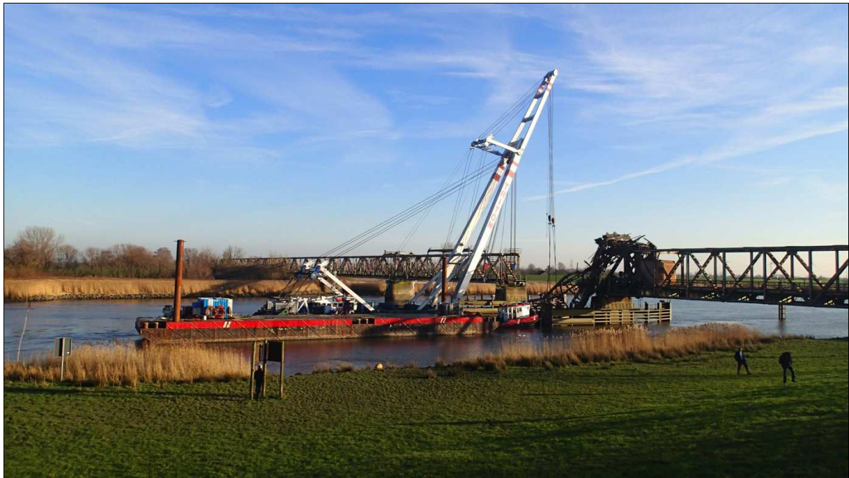
Figure 3: Recovery of the bascule
