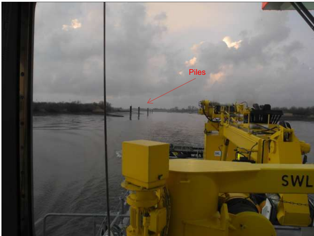
Figure 24: Piles for the shipping
