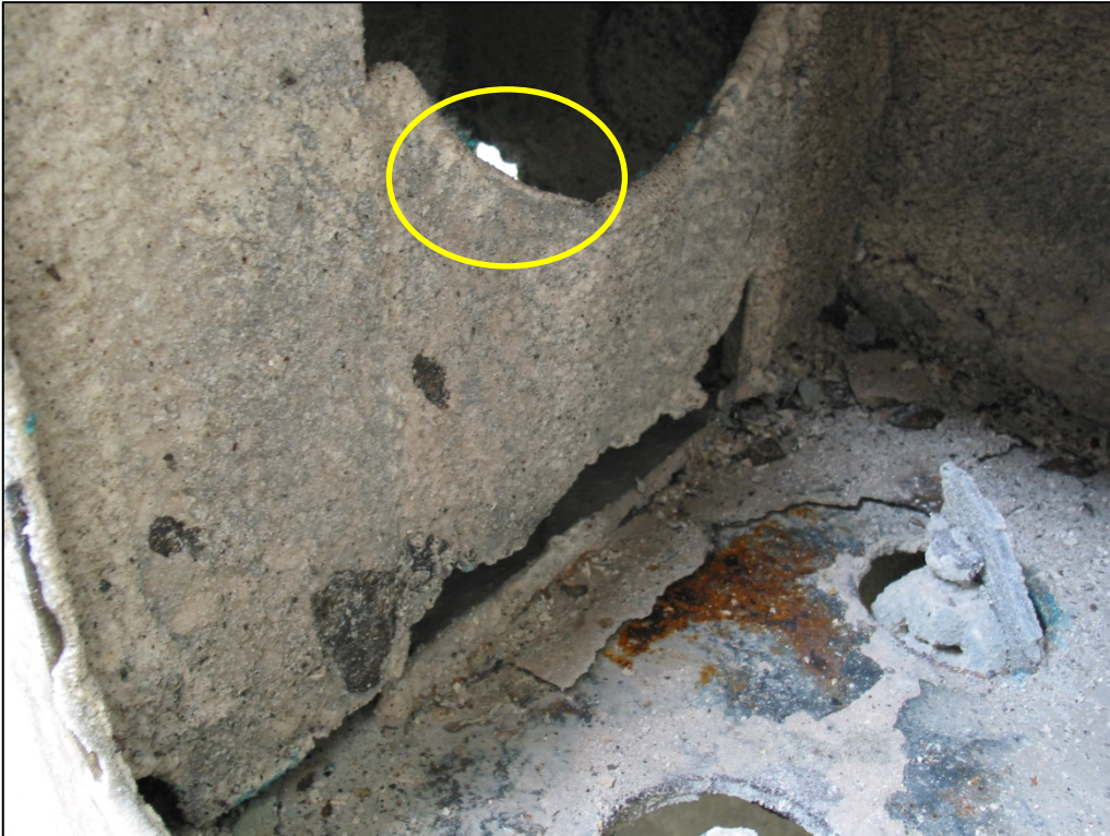
Figure 36: View in the opening to void space A and B
