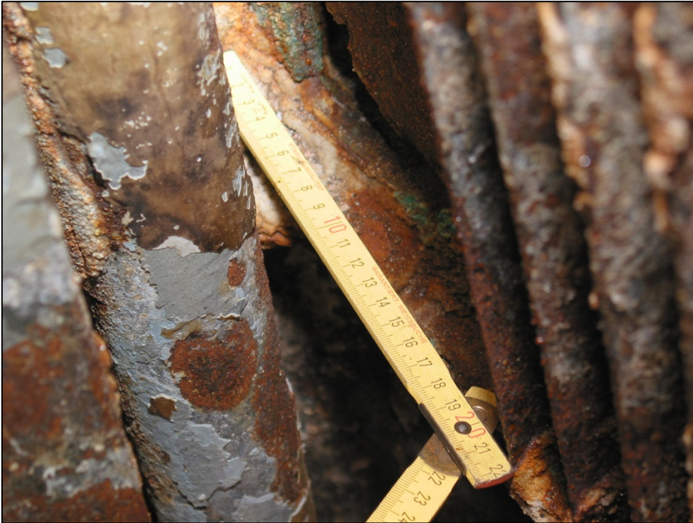
Figure 60: Hold ladder trunk to cargo hold 2
