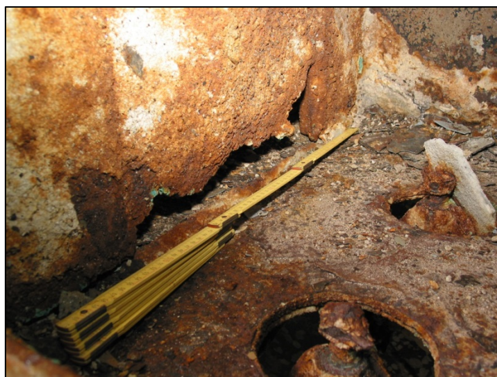
Figure 59: View in the void space A (see also image 36)
