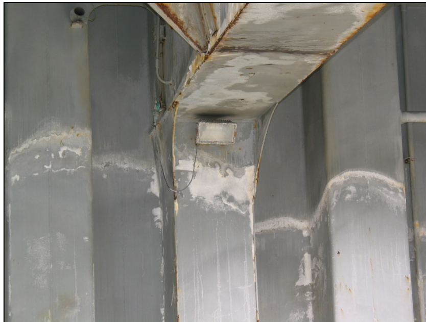
Figure 46: Cargo hold 4, lower hold, aft cargo hold light
