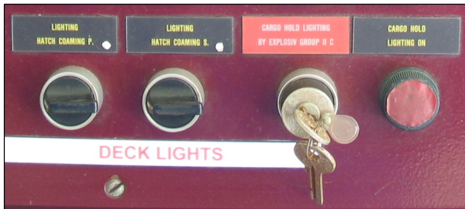
Figure 25: Master switch for the cargo hold lighting on the bridge
