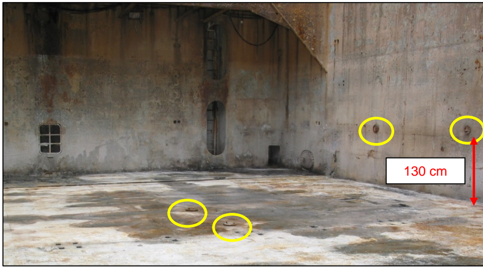
Figure 27: Additionally mounted D-rings
