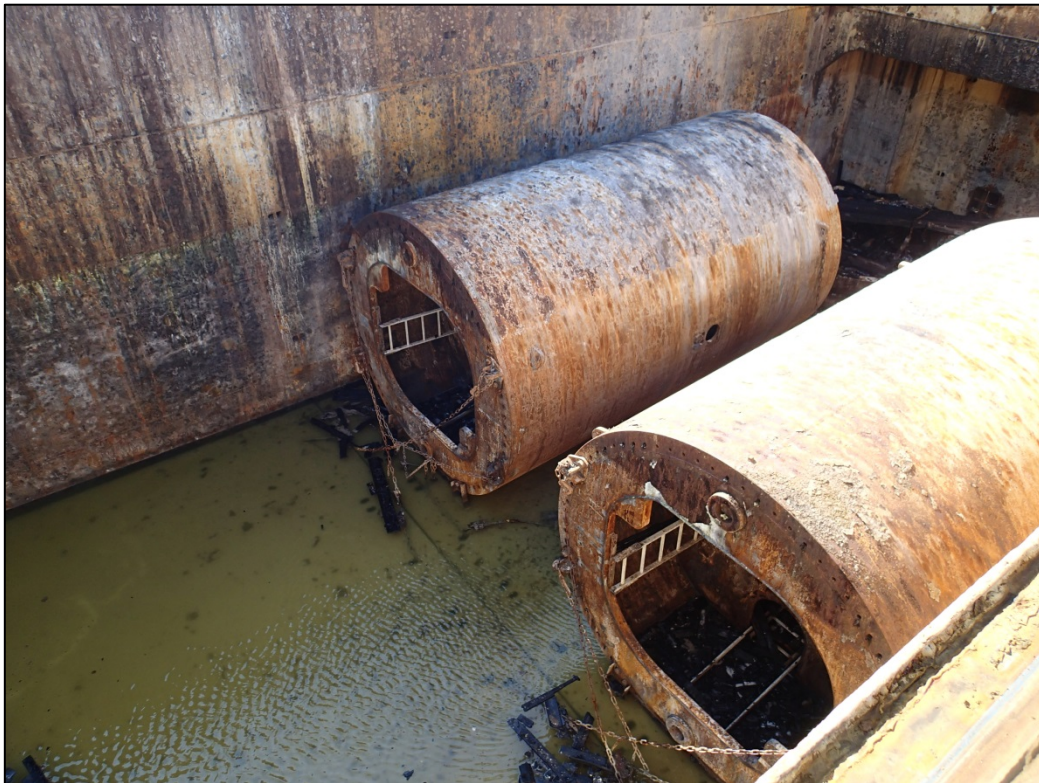
Figure 14: Cargo hold 3, tween deck, port side, 5 June 2015
