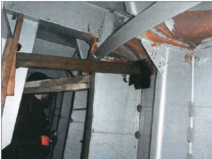
Figure 21: ...with water ingress
