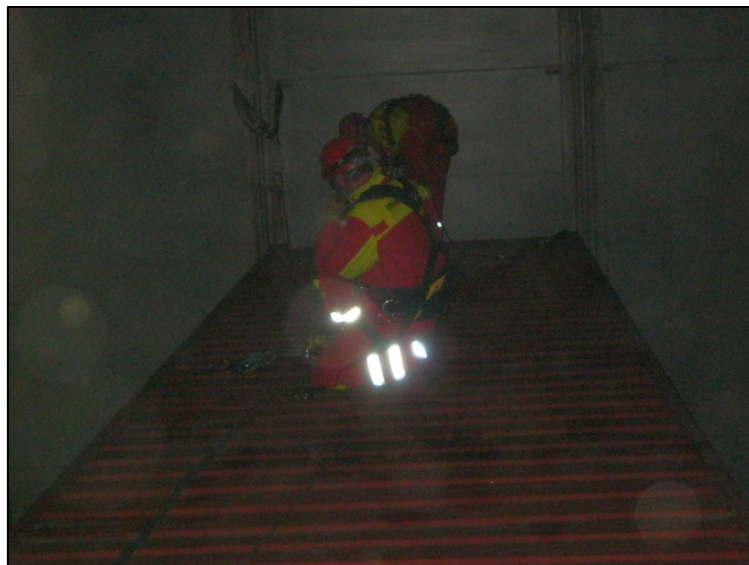
Figure 13: Erecting safety equipment on the roof of the uppermost container
