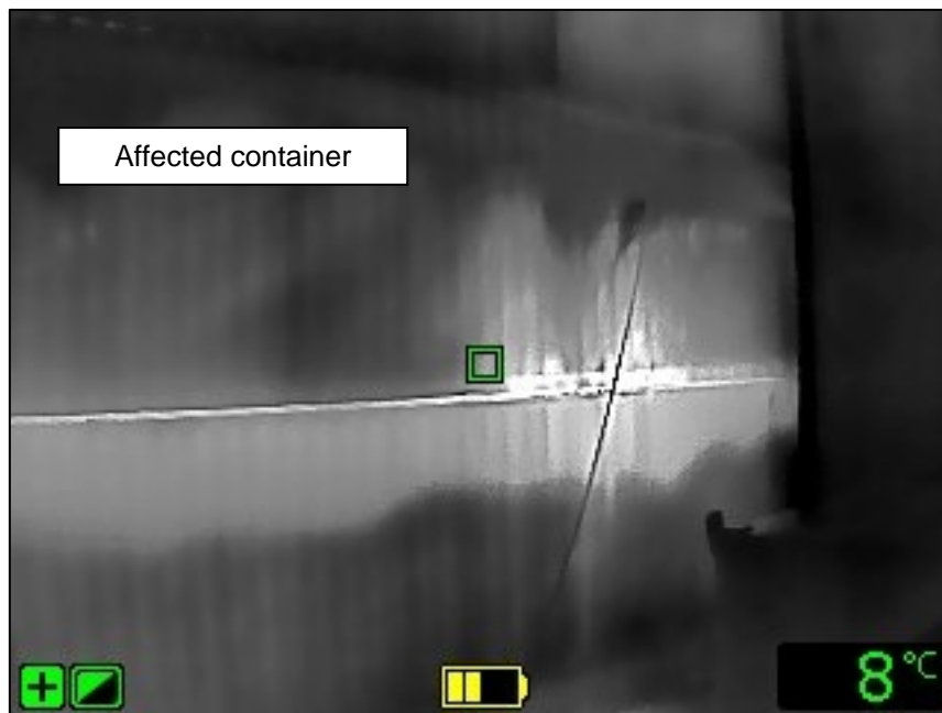
Figure 15: Temperature measurement by the fire service on the starboard side of the stack: 8 °C
