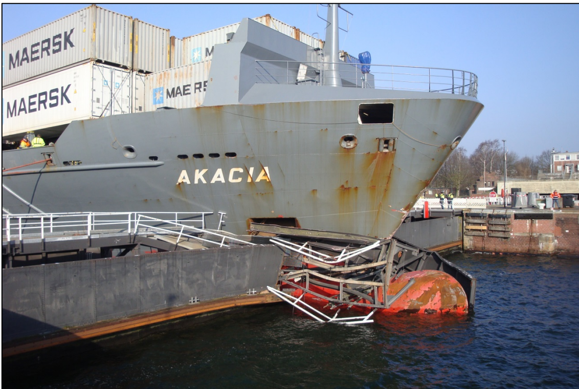
Figure 4: The AKACIA and the damaged lock gate
