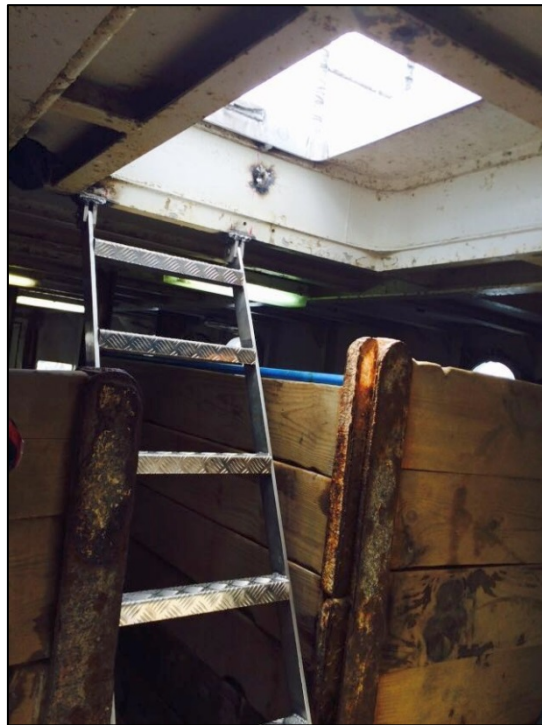
Figure 24: New means of accessing the observation deck seen from below
