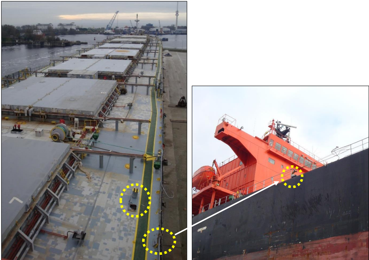
Figure 10: Positions of the destroyed bollard and broken hawsehole
