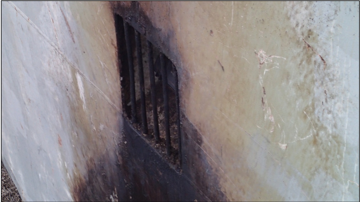
Figure 6: Fire damage on the starboard leading edge of cargo hold 1
