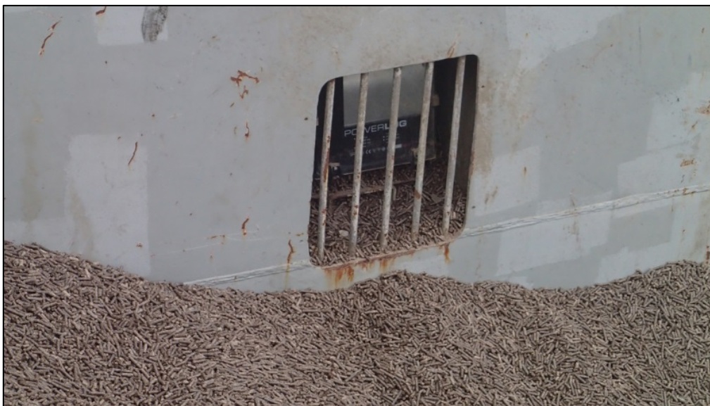
Figure 14: Port cargo hold light
