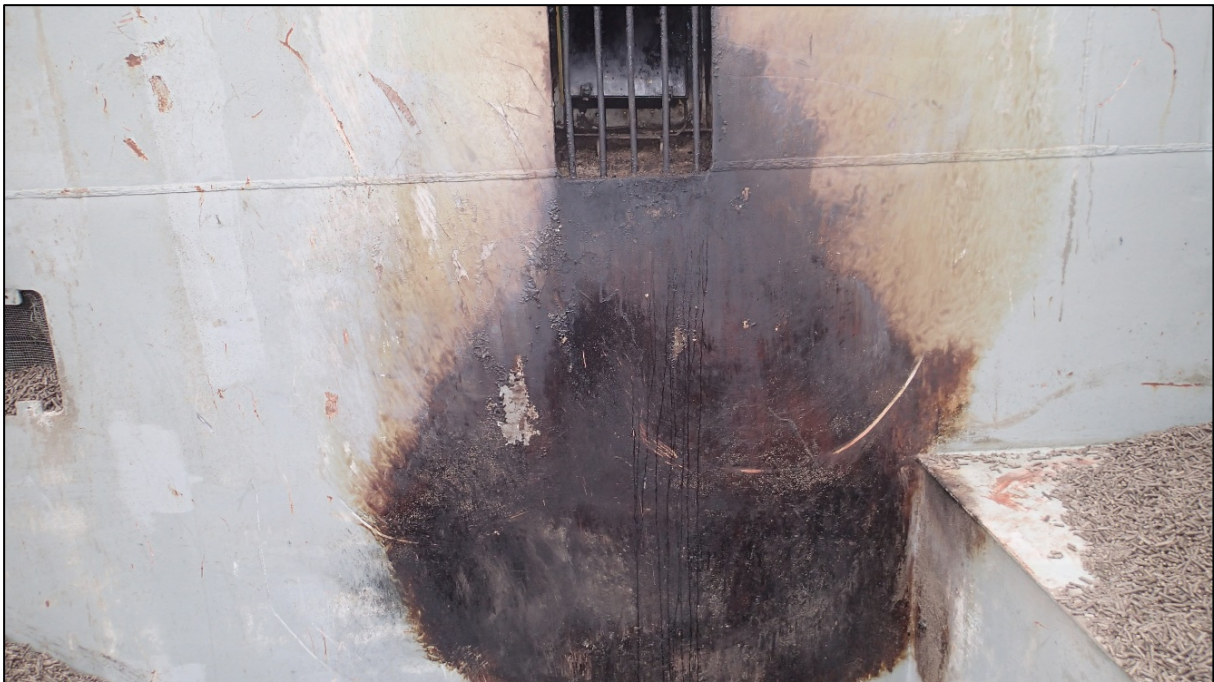
Figure 8: Smouldering fire range up to 2 m below the cargo hold light
