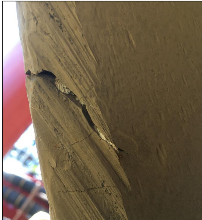
Figure 38: Crack in one of the propeller blades Remnants of line were found in the crack.
