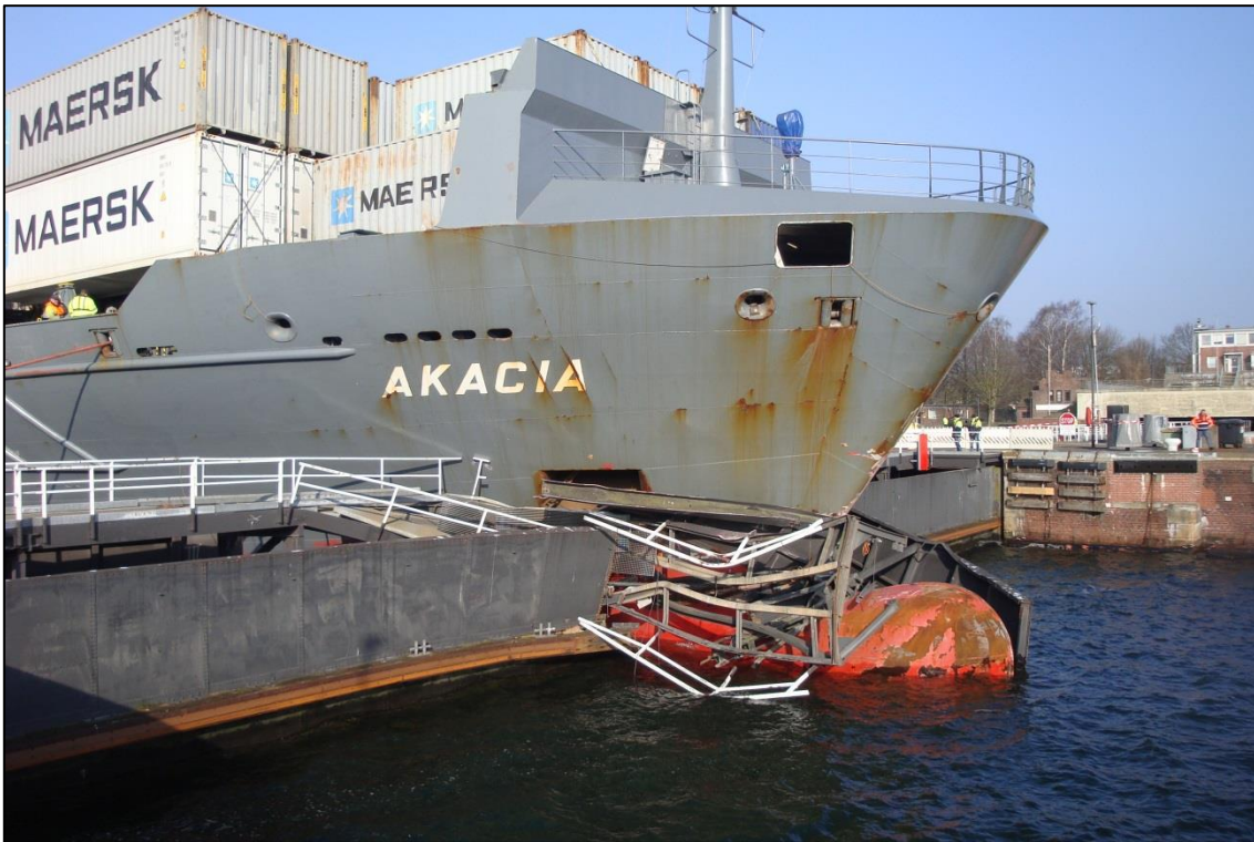
Figure 4: The AKACIA and the damaged lock gate
