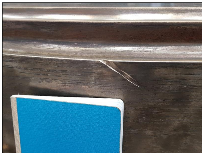
Figure 53: Notch on the bearing plate
