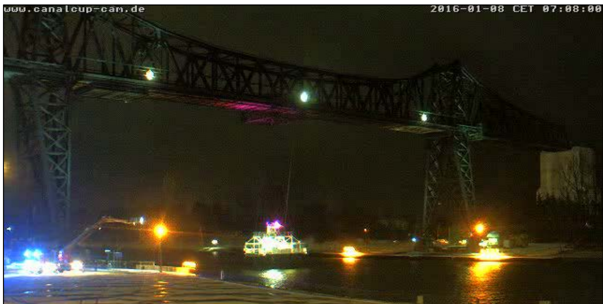
Figure 14: Start of the rescue operation by the fire service (08/01/2016, 0708)
