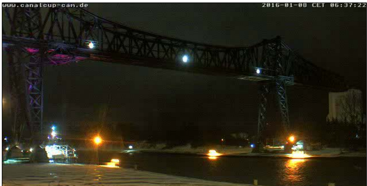
Figure 8: Bridge lighting on the northern bank is turned off (08/01/2016, 0637)
