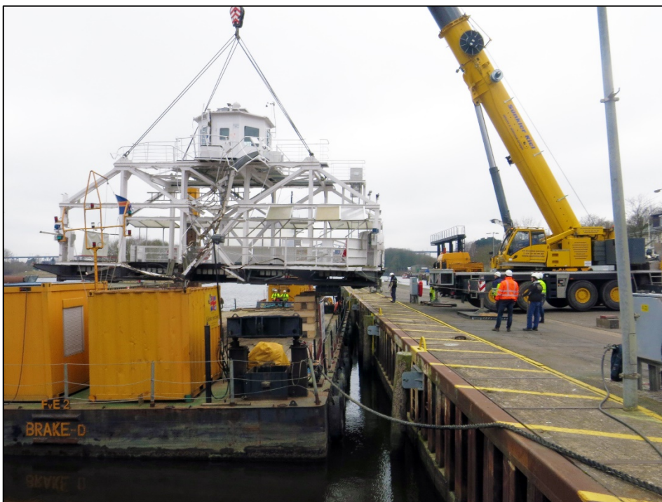
Figure 22: The transporter bridge being unloaded at the WSA's dockyard
