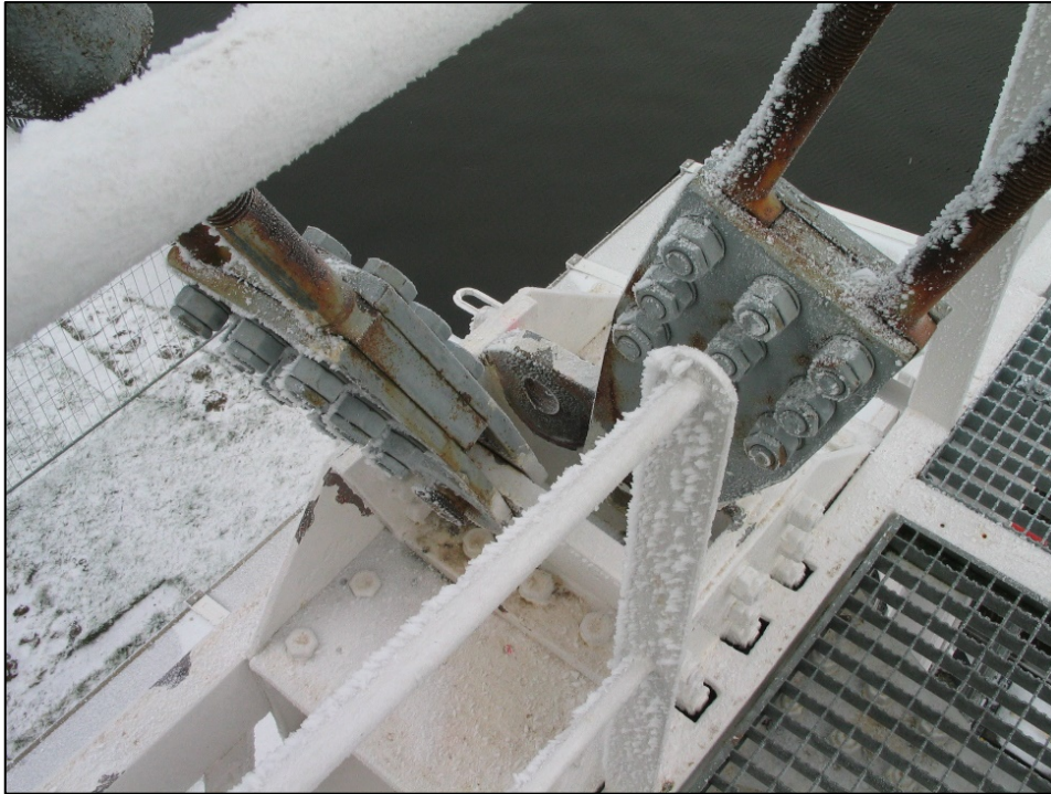
Figure 43: Cable attachment point on the north-western side
