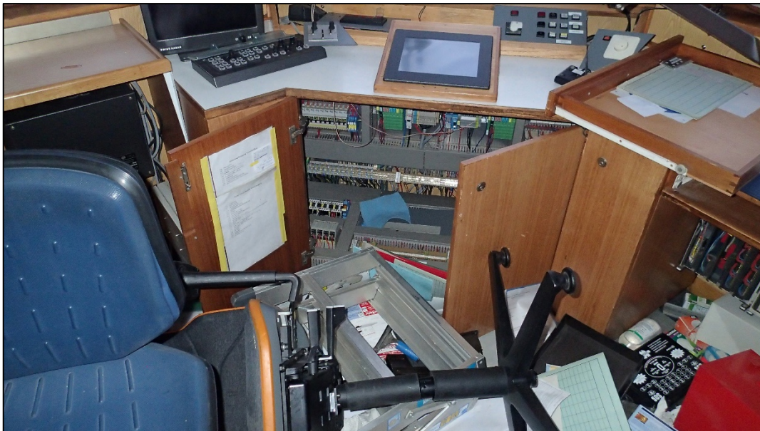
Figure 44: View into the control position from the door
