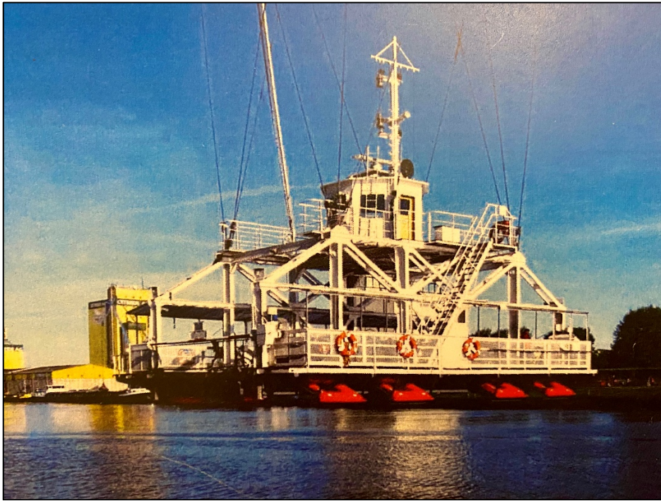
Figure 72: Transporter bridge before the accident – view from the direction of the EVERT PRAHM
