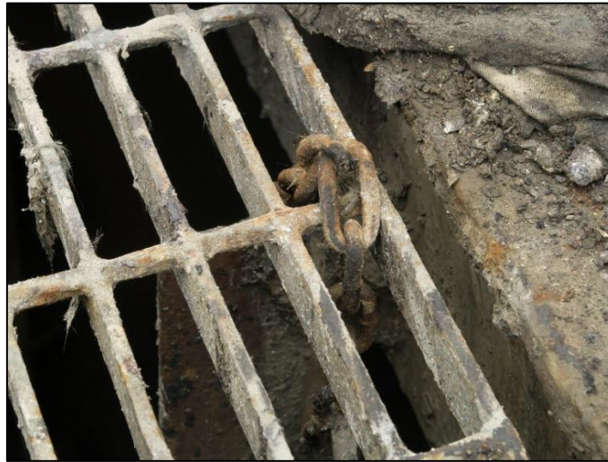
Figure 55: Grill over ventilation opening secured by chain and lock
