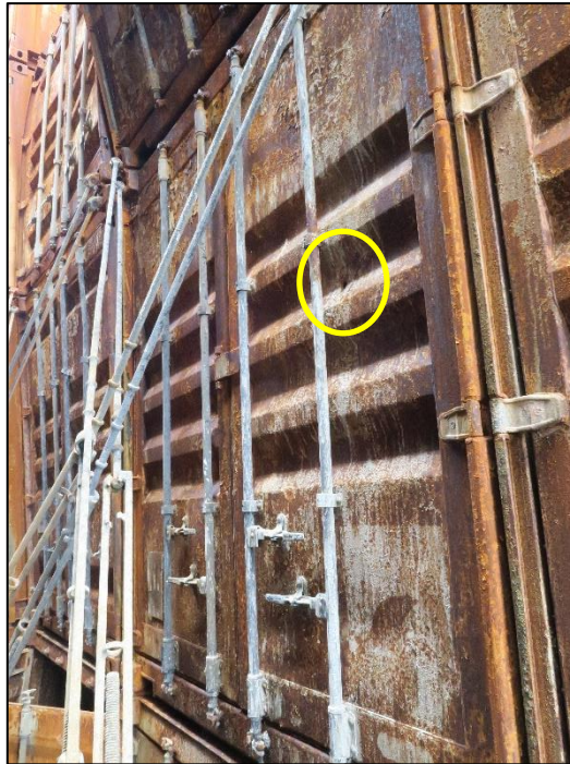
Figure 57: Container at slot 120984 with hole for water mist lance
