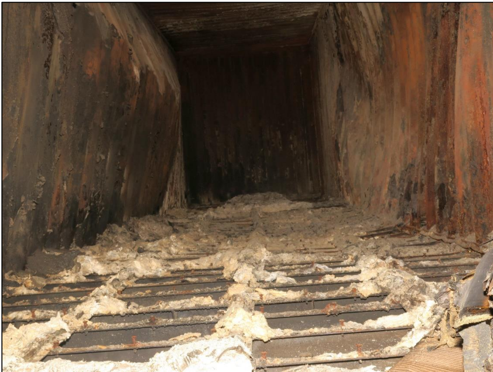
Figure 29: View into the container at slot 120382
