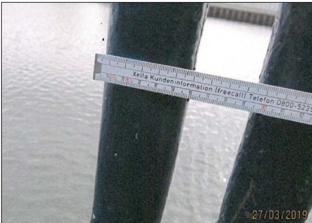
Figure 6: 6 cm diameter handrail
