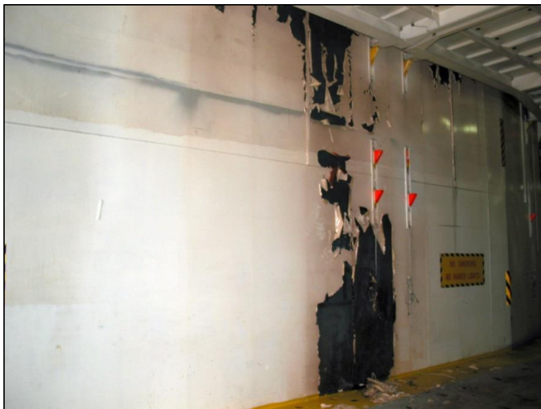
Figure 11: Damage to the paint coating
