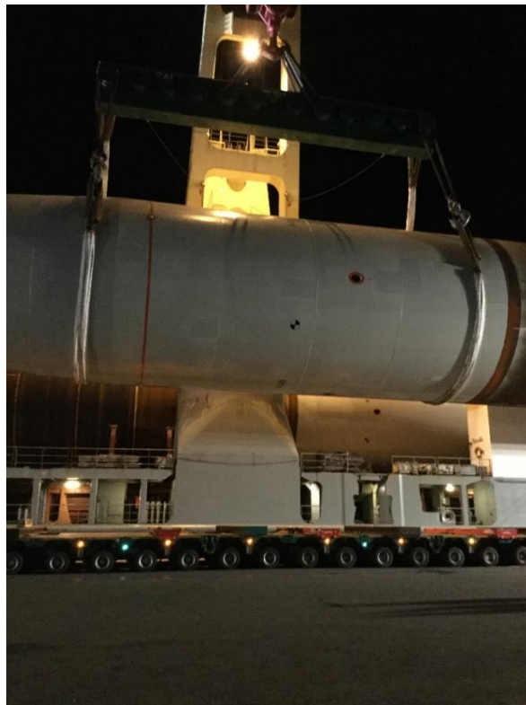
Figure 10: Lift before the swing operation
