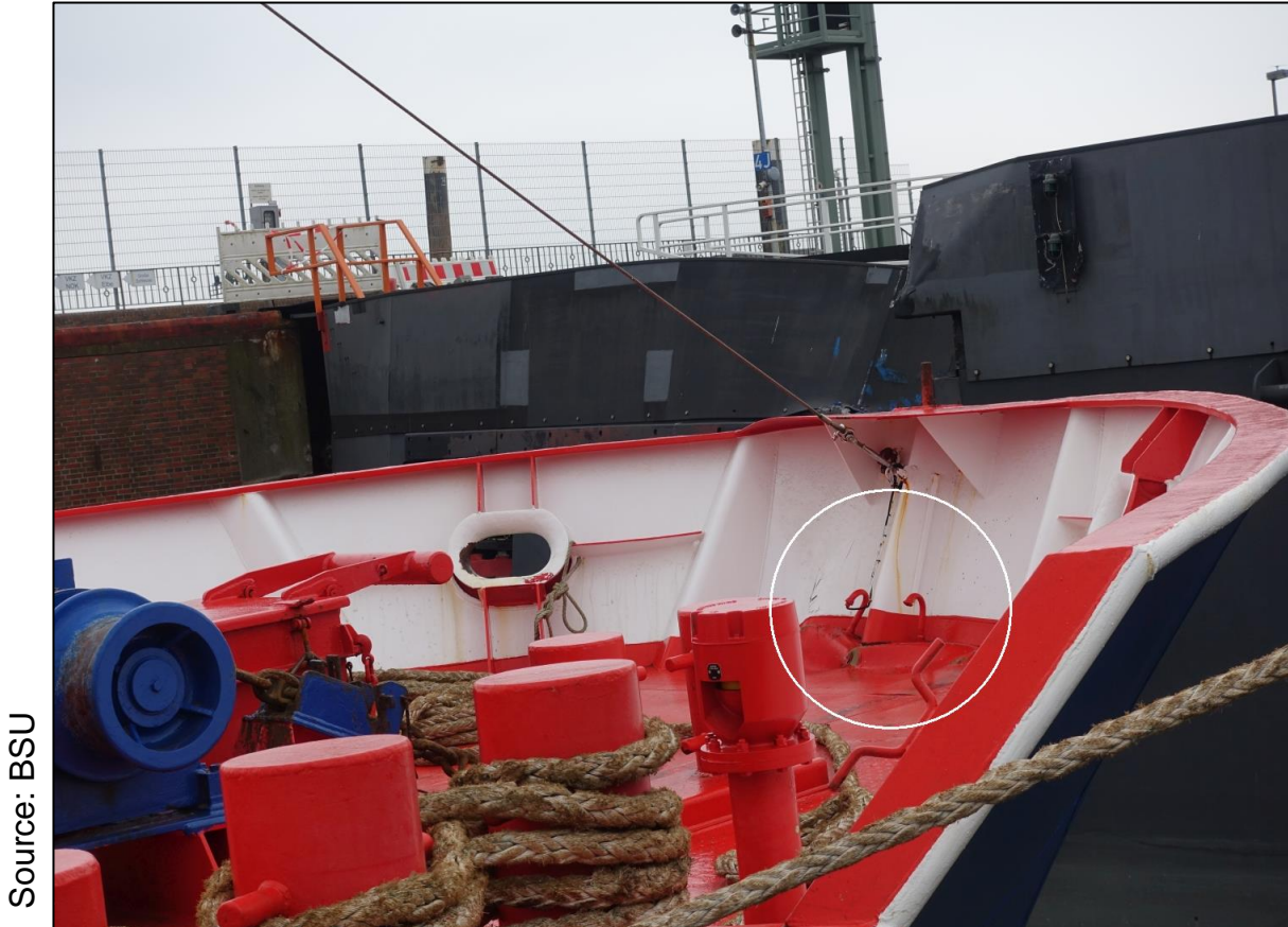
Figure 5: Deformed deck plating in way of forecastle
