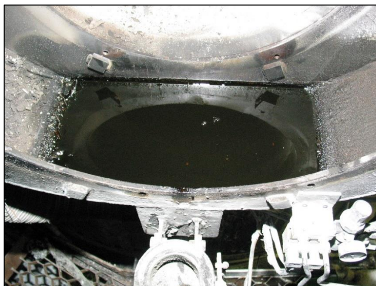
Figure 17: Fuel in the windbox
