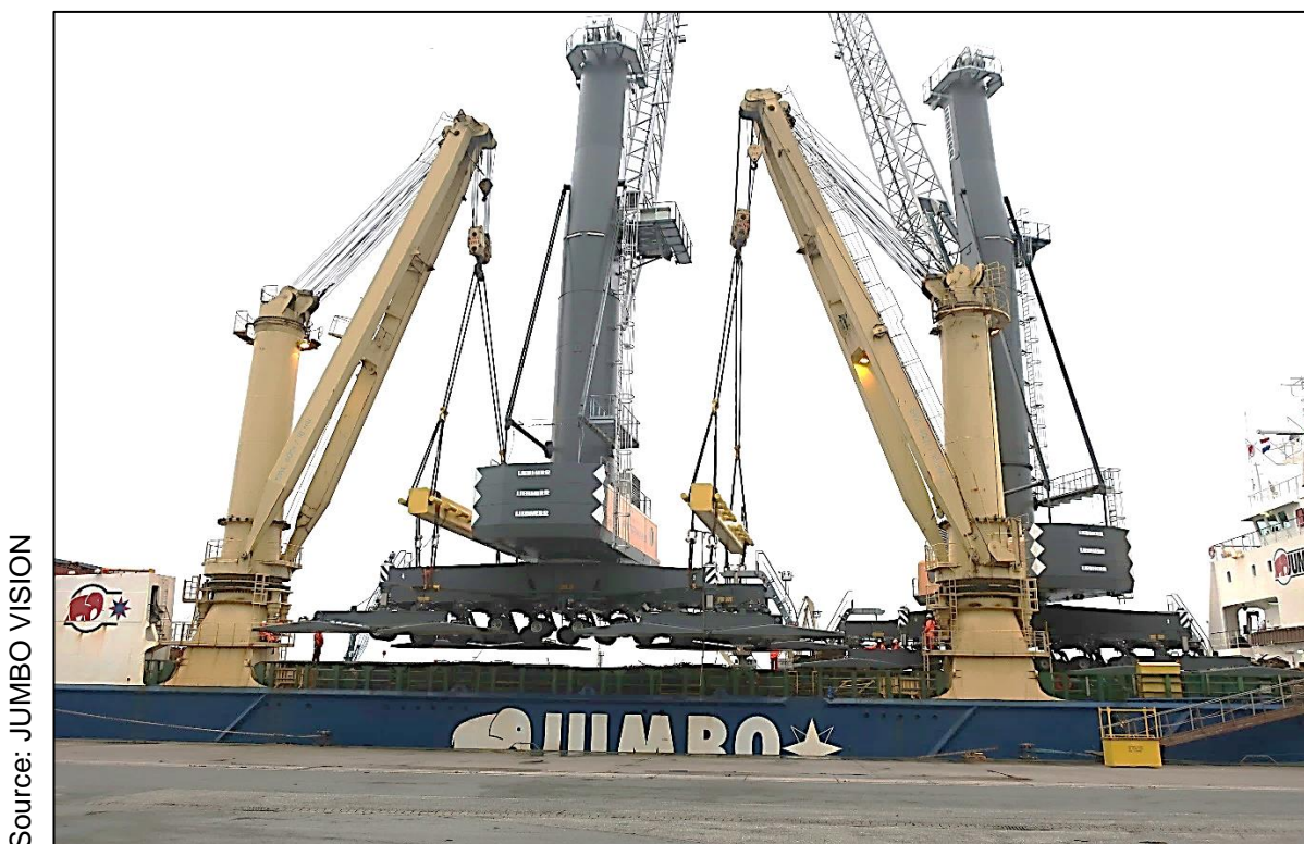
Figure 6: Crane 2 being tandem lifted
