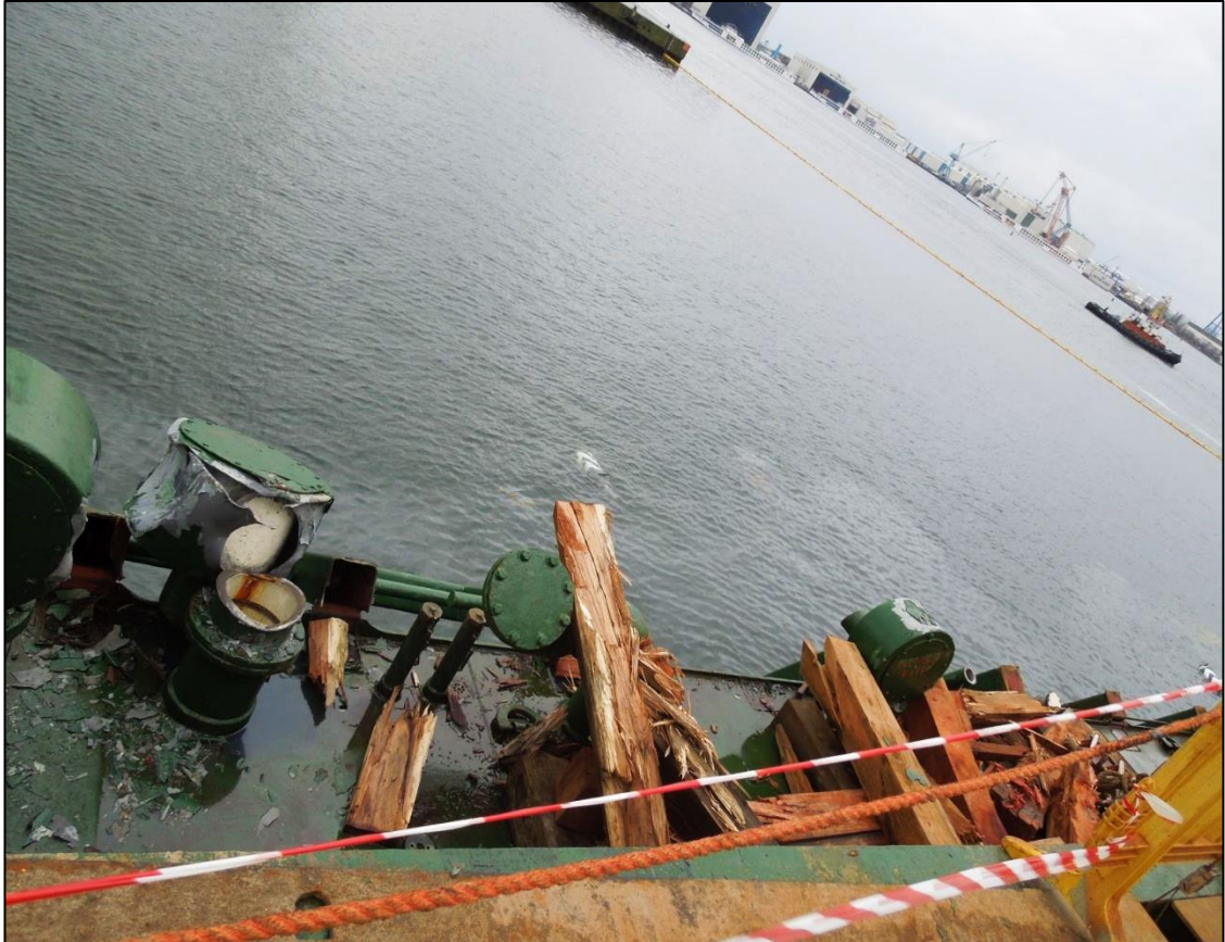
Figure 13: Damage to port-side deck passageway caused by crane 2 (sounding pipes, vent heads, overflows, wooden blocks, missing railing)
