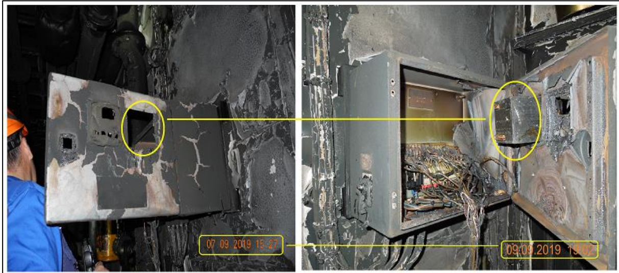
Figure 13: Alterations to the control cabinet
