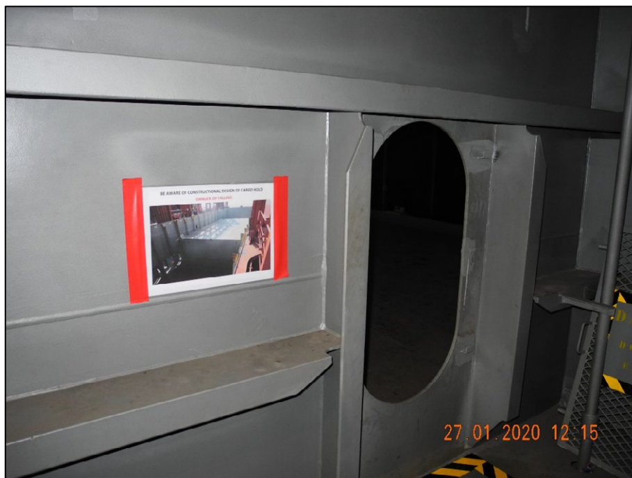
Figure 28: Photograph showing the actual Risk of Falling 80
