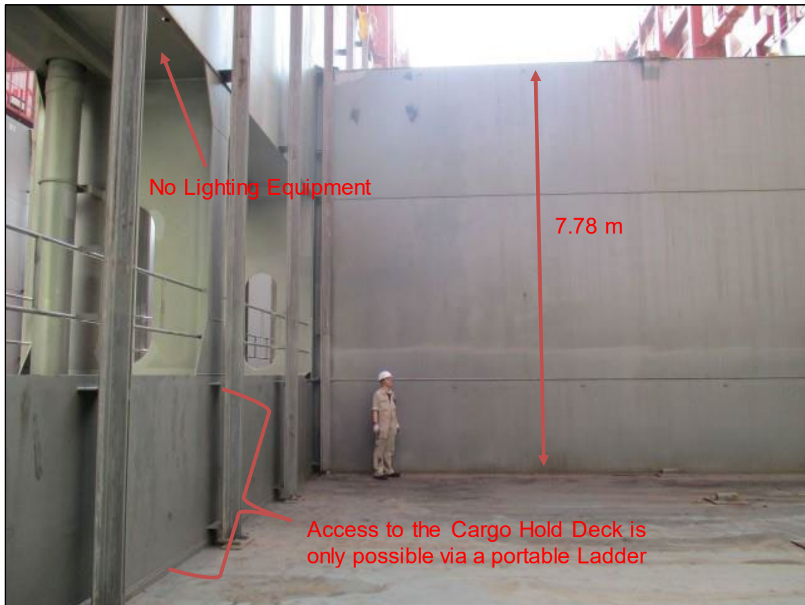
Figure 8: Height of Fall, Lack of Lighting, Access to the Cargo Hold Deck 20
