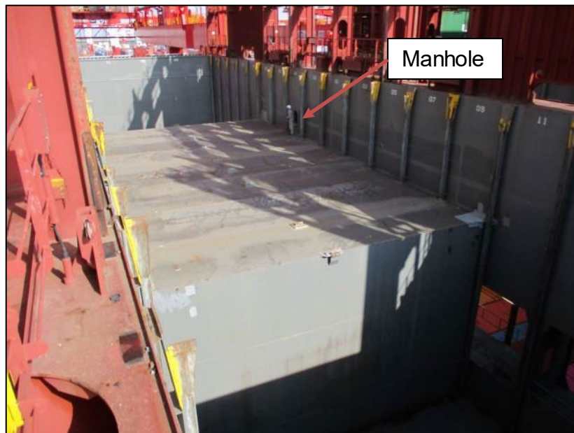
Figure 6: View of the Enclosure from the Starboard Side with open Hatch Cover 18
