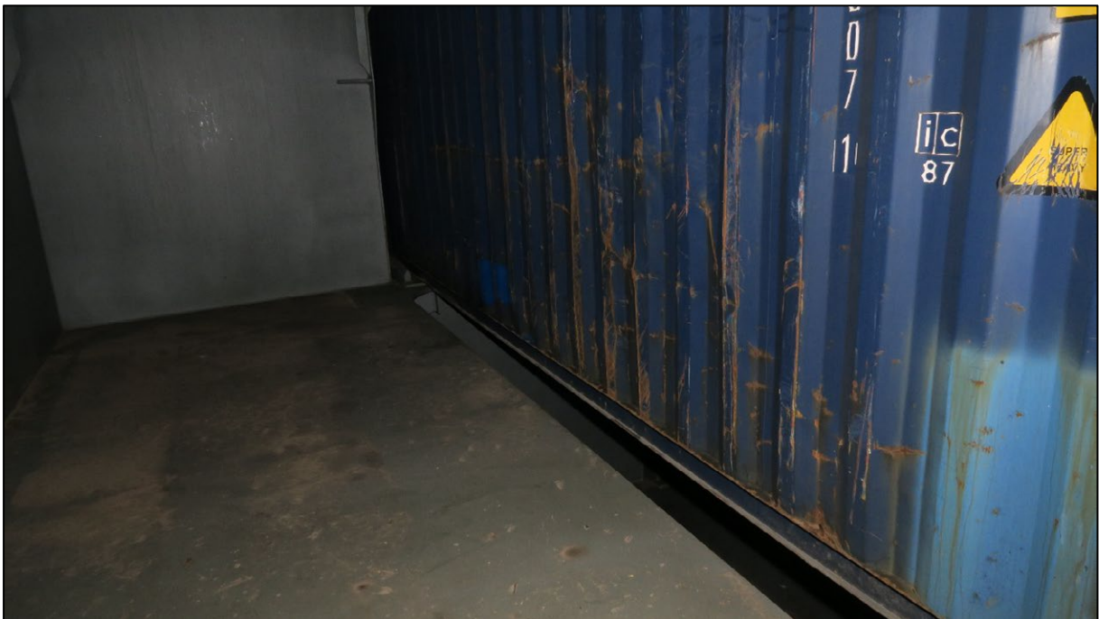
Figure 30: Area that has yet to have Fall Protection applied 82
