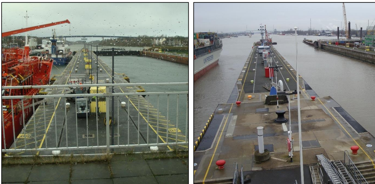
Figure 17: Edge marking on the lock walls in Kiel-Holtenau (left) and Brunsbüttel (right)
