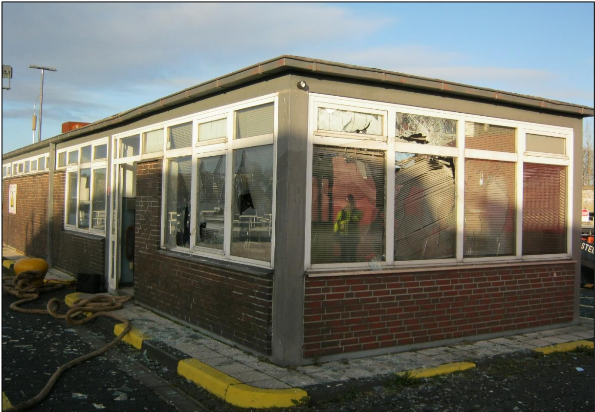
Figure 4: Service building (close-up of the affected part of the building)
