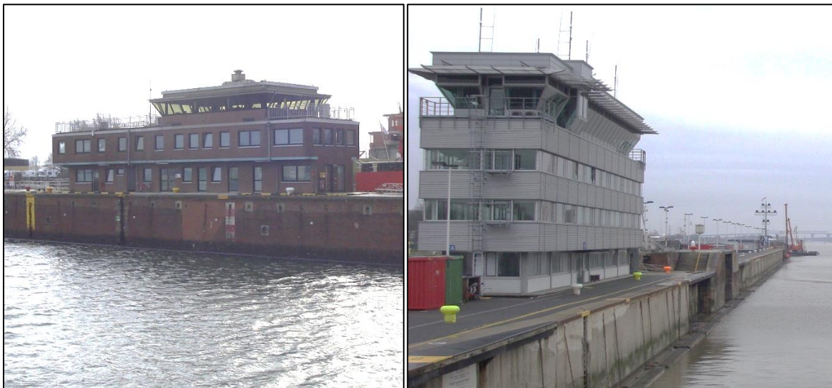
Figure 18: Lock control stations in Kiel-Holtenau (left) and Brunsbüttel (right)
