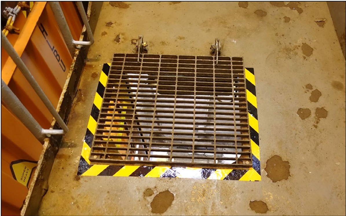
Figure 19: Yellow and Black Markings on a Deck Passageway 115
