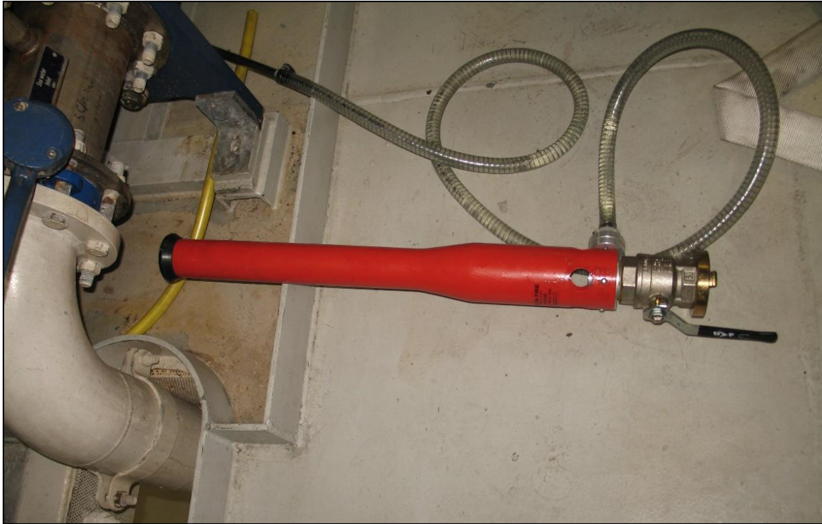
Figure 27: Mobile low-expansion foam pipe with integrated inductor
