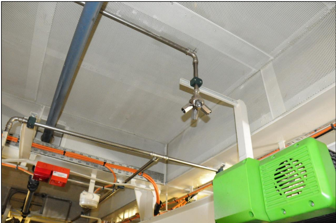
Figure 30: Room protection system
