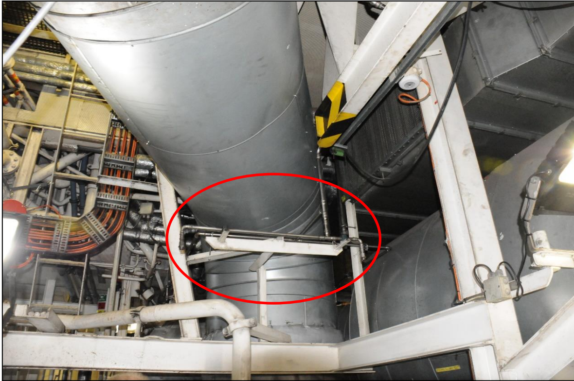
Figure 38: Object protection turbocharger area
