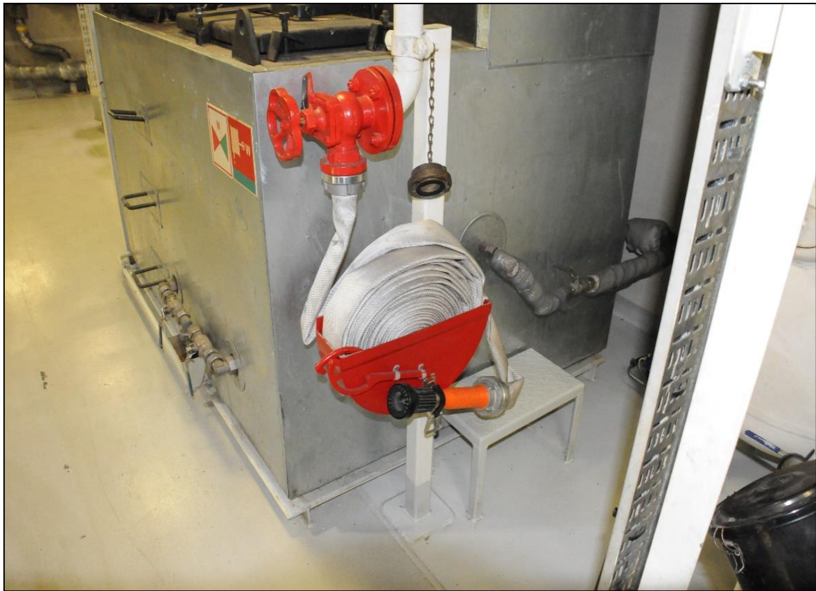
Figure 25: Standard jet pipe / hydrant system
