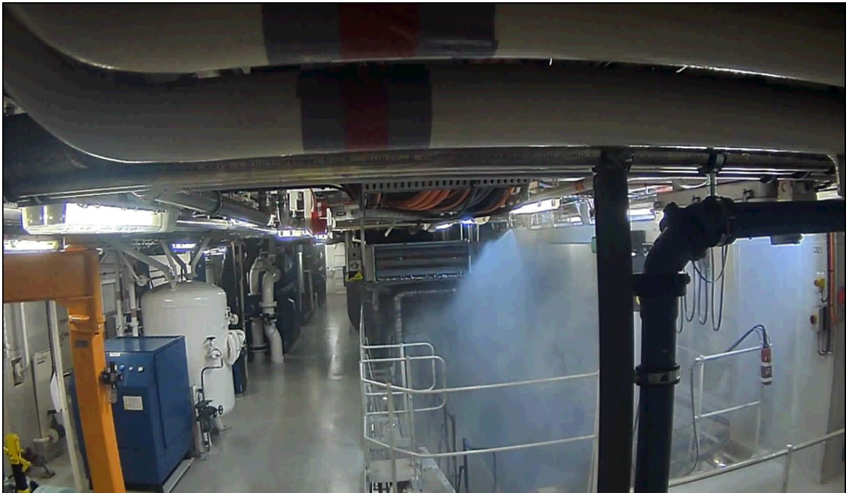
Figure 5: Object protection system triggered above ME 3 10
