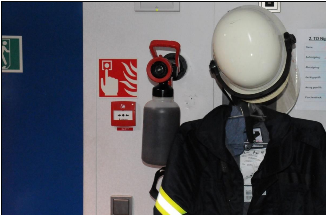
Figure 34: Venturi turbo jet pipe with 2 ltrs. of F-500 EA, for flexible initial attack in all engine-room areas, positioned in the Engine Fire Locker (firefighting equipment room)
