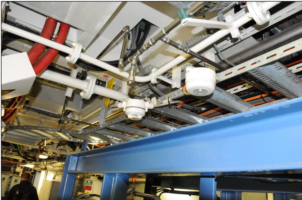
Figure 28: Object protection system
