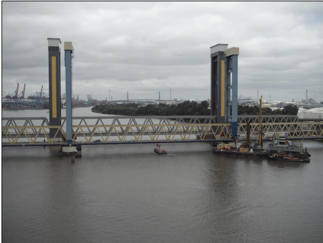
Figure 4: The Kattwyk bridge, which was also lowered at the time of the accident 3
