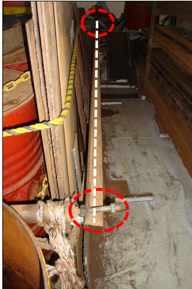
Figure 4: Stack of plates 4 secured by a steel cross strut
