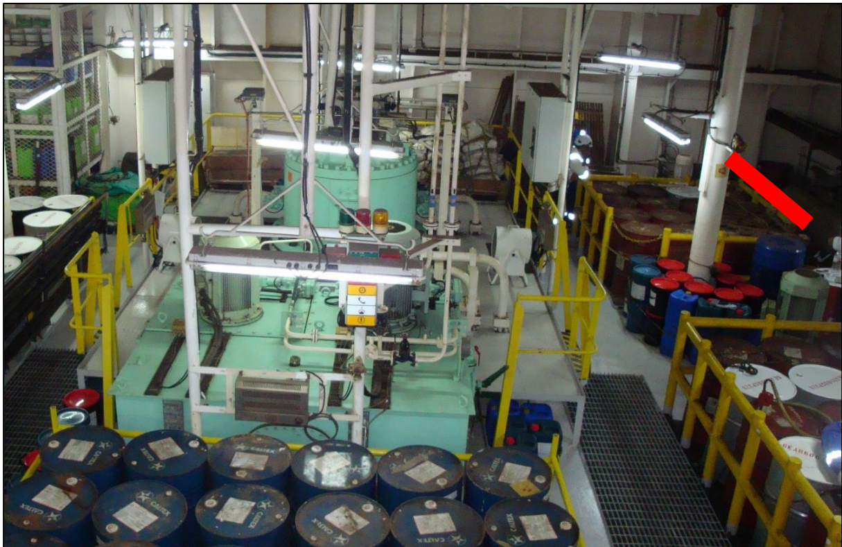
Figure 3: Steering gear room (Site of the steel plates marked red)
