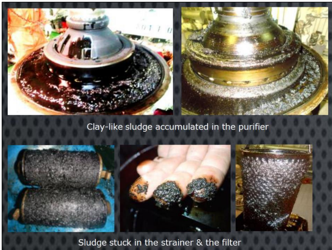
Figure 13: Oily sludge in purifiers and filters after fuel blending 48 (precipitated asphaltenes)
