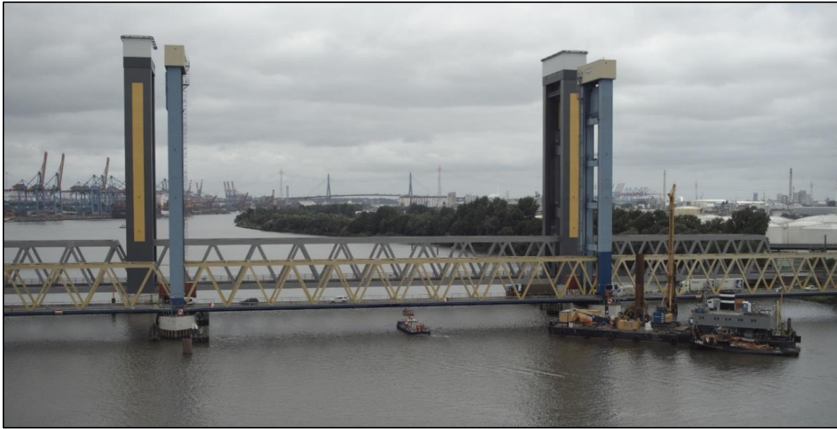
Figure 17: The Kattwyk bridges, which were also lowered at the time of the accident. 21
