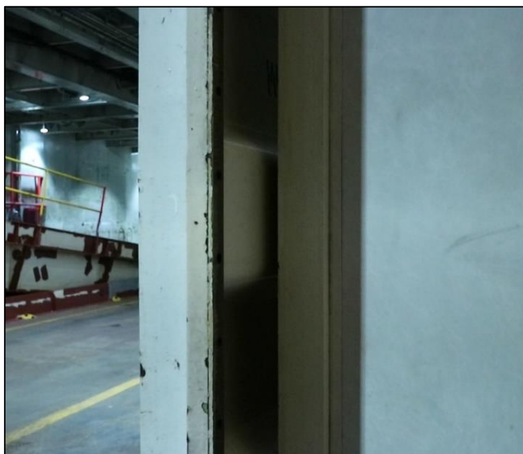
Figure 12: Watertight door number 110 when it is opening 15
