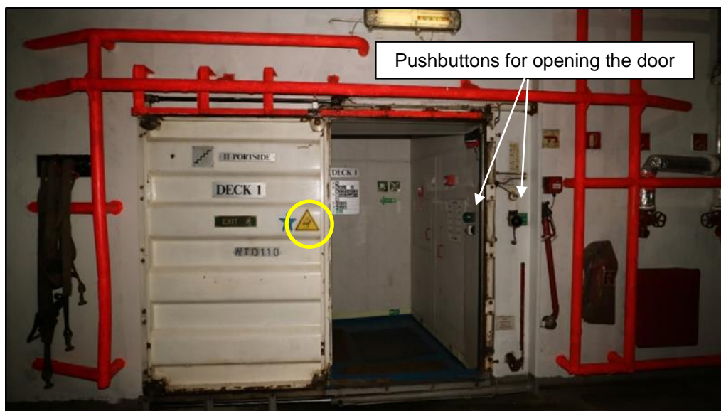
Figure 4: Watertight door number 110 on deck 1 in the open condition 7 The yellow circle marks the warning sign indicating a risk of crushing.
