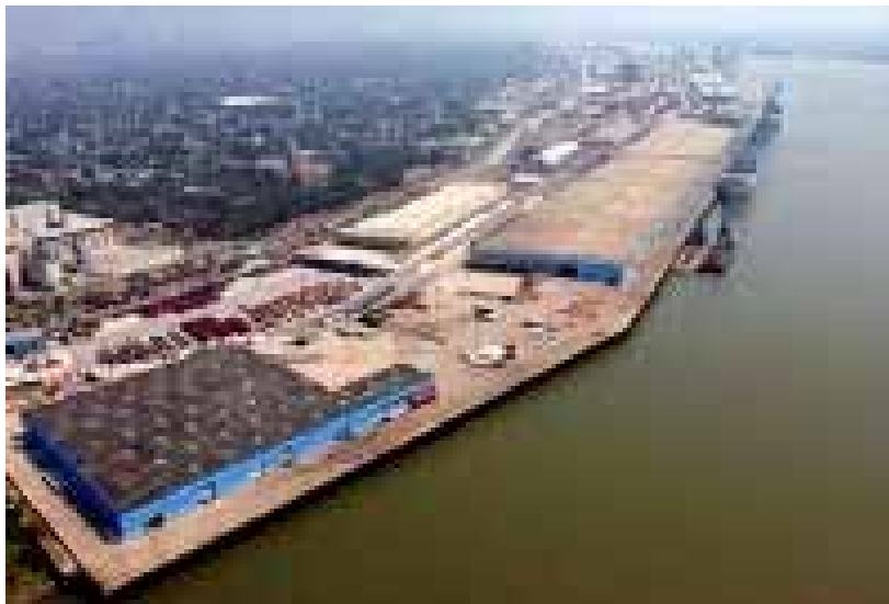
Figure 2: Aerial photo of the port facility
