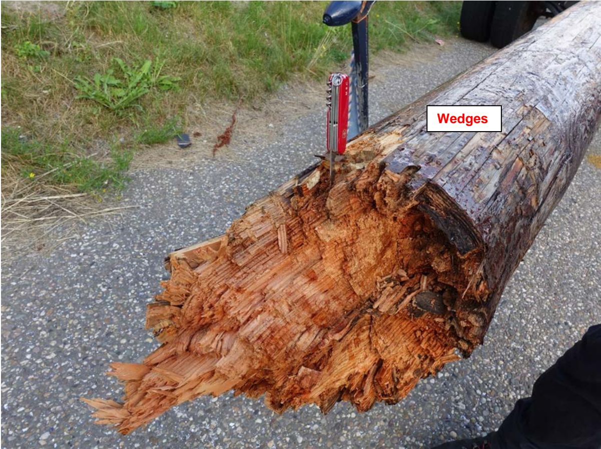
Breaking point on the remaining part of the mast.
